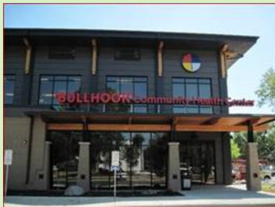
Bullhook Community Health Center, Havre, MT Photo Credit: Bear Paw Development Corporation
