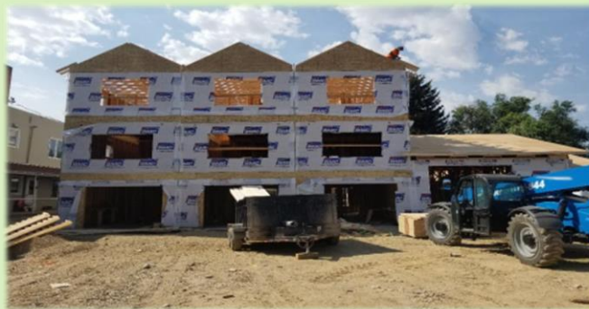
Figure 2: Construction has begun at the Lee Gordon Place
