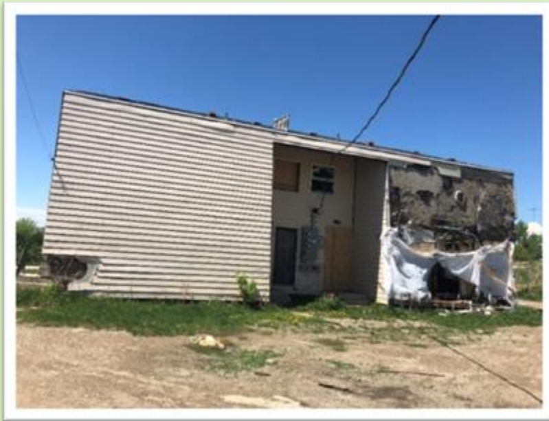
Figure 2: One of the original L'BelCour Housing Structures.
