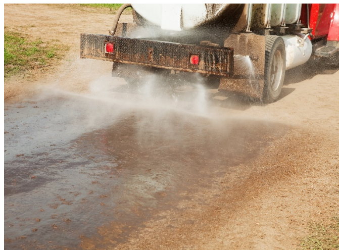
A truck applies chemical stabilizers to a roadway for dust suppression.
