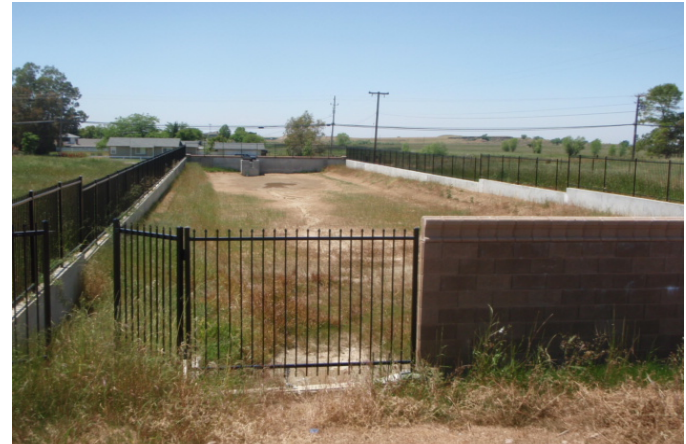
Dry detention pond with security fencing. Credit: Jared Richardson for USEPA, 2012
