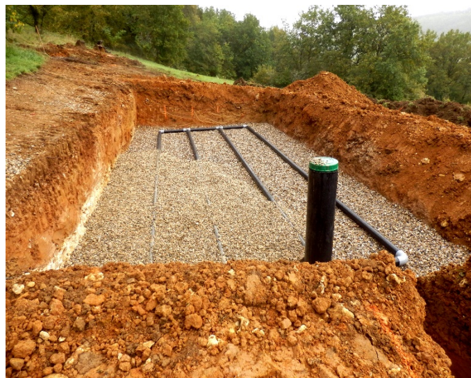
A sand filter under construction.
