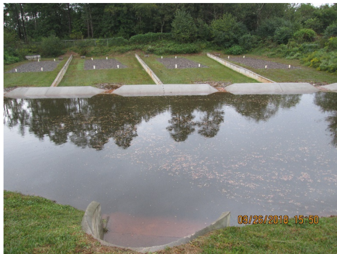
Water flows from a stormwater inlet into the pre-treatment basin of a sediment chamber, then overflows through weirs into four separate gravel sediment filters.
