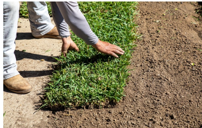
Sod can be used to quickly stabilize soil and reduce erosion
