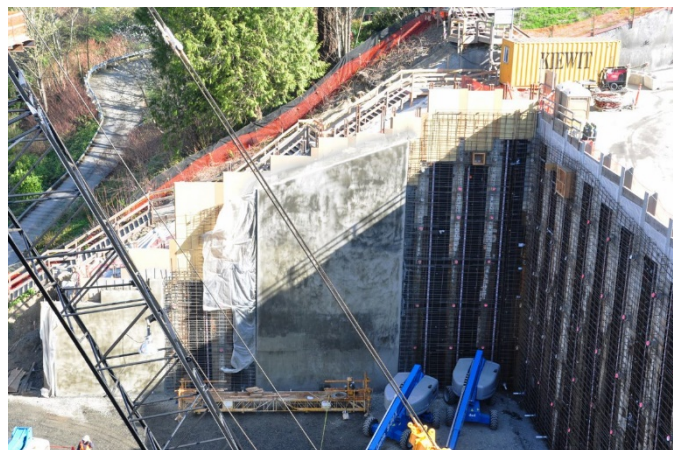
A retaining wall supporting soil along a steep slope.
