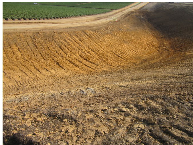
Soil roughened with tracked machinery can provide temporary erosion control.
