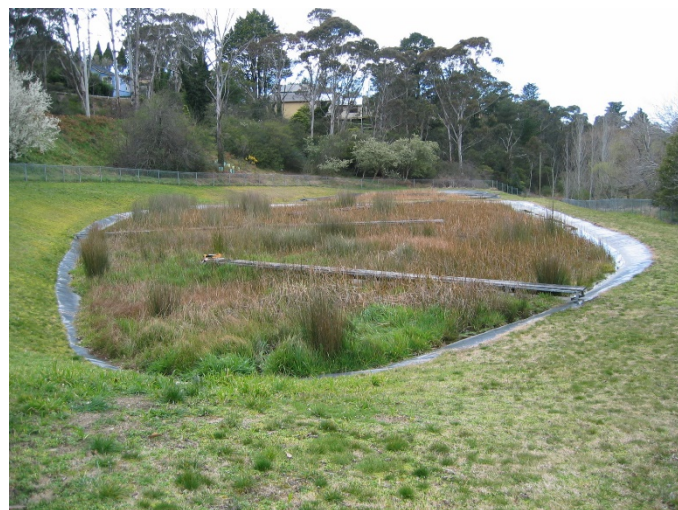
Stormwater wetlands provide a reduction in stormwater pollutants as well as provide wildlife habitat.
