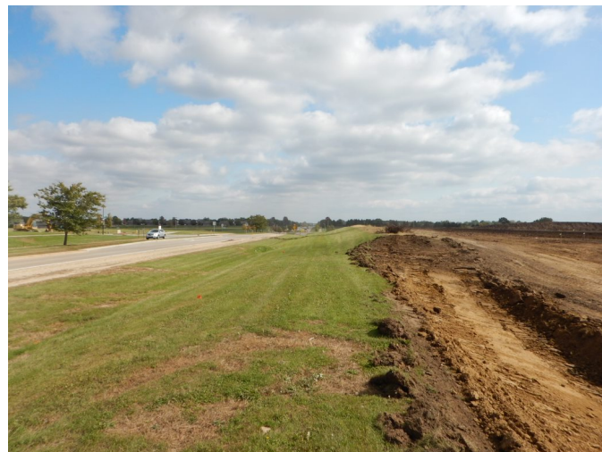
Using a vegetated buffer along the perimeter of a construction site can deter sediment from moving off site.
