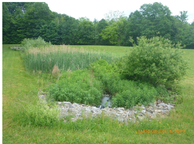
A vegetated filter strip can infiltrate and treat stormwater flow from adjacent surfaces using a variety of plants.
