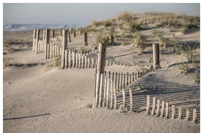
A wind fence that has trapped sand along a beach dune.
