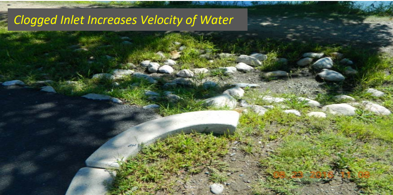
Water Overtops Containment Berm
