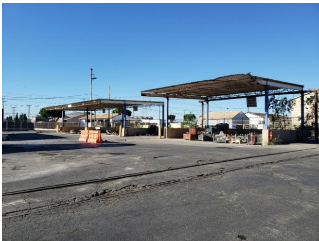
Container Storage Areas Decontamination and Deconstruction
