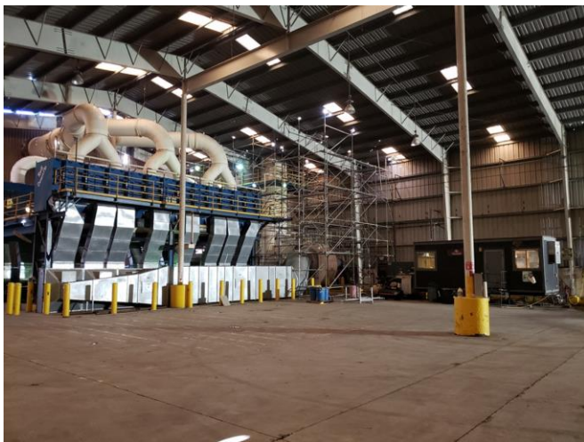
Torit Baghouse Units Decontamination and Deconstruction
