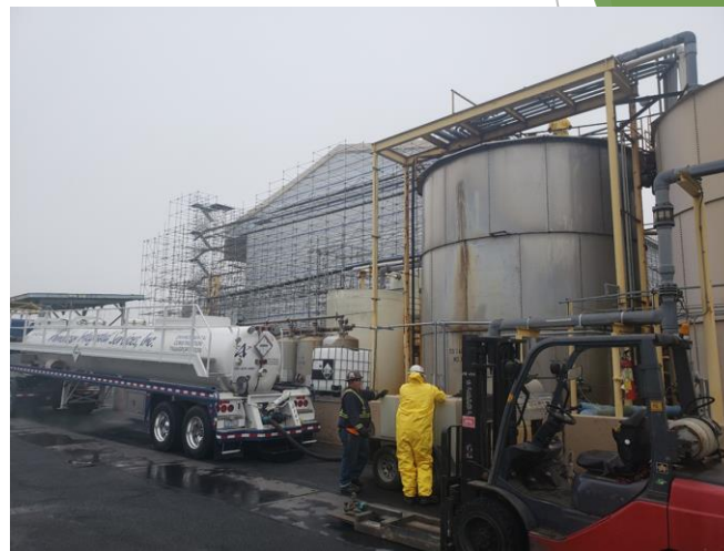
WWTP Tank Clean- outs
