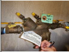
11: DSCN0352JPG Location: Benton Harbor PWS Photographer: Naomi Huff Date/Time: 9/21/2021 9:38 AM
