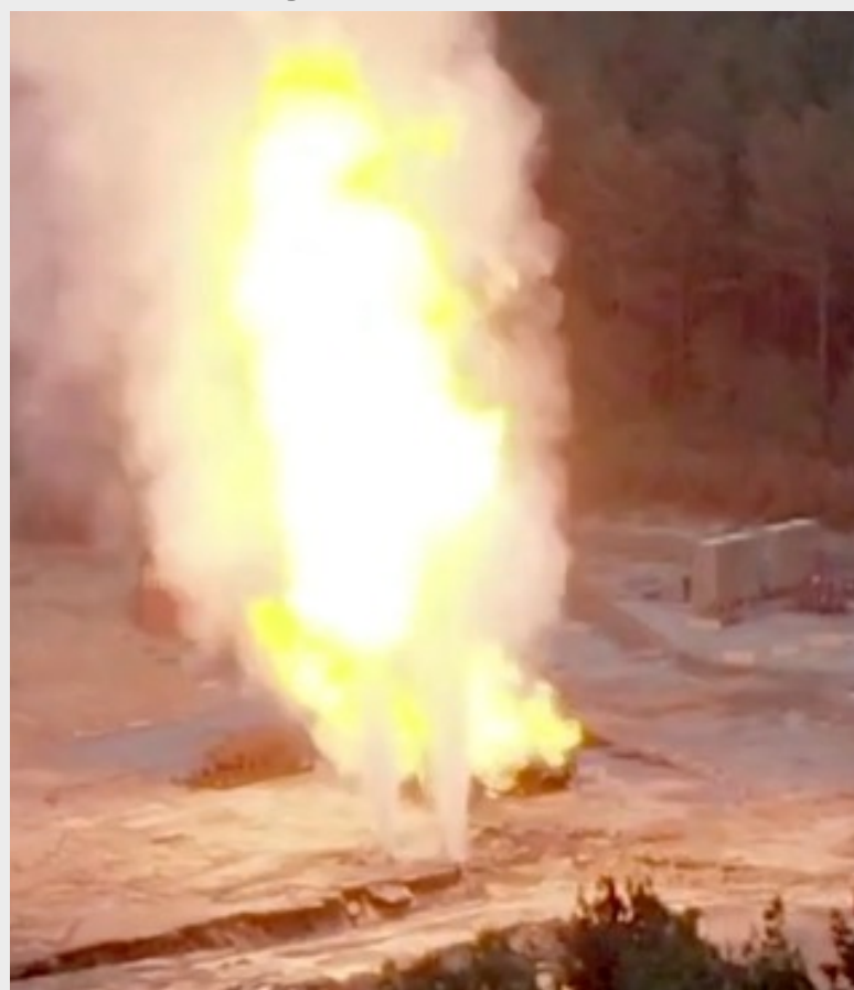
Venting at the wellhead
