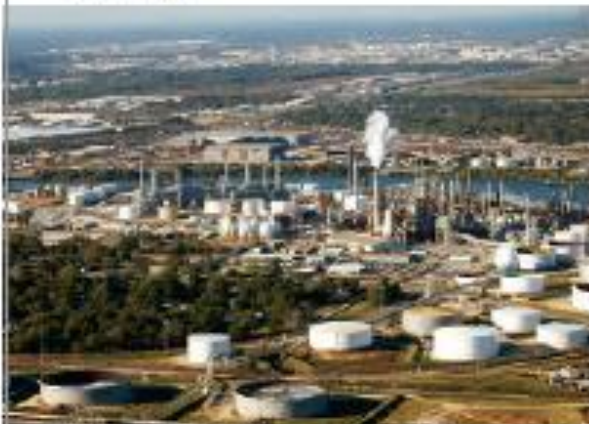
Houston contains 191 high-risk chemical facilities.
