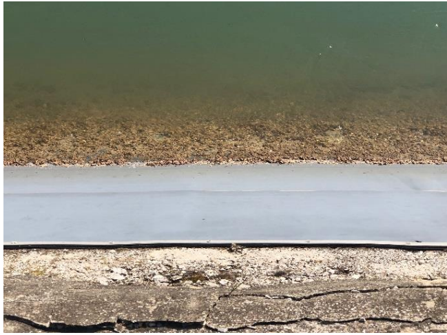
Benthic mats on canal walls, (a waterproofing membrane is used in this part of canal)
