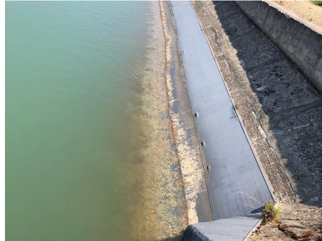
Benthic mats on canal walls, (a waterproofing membrane is used in this part of canal)
