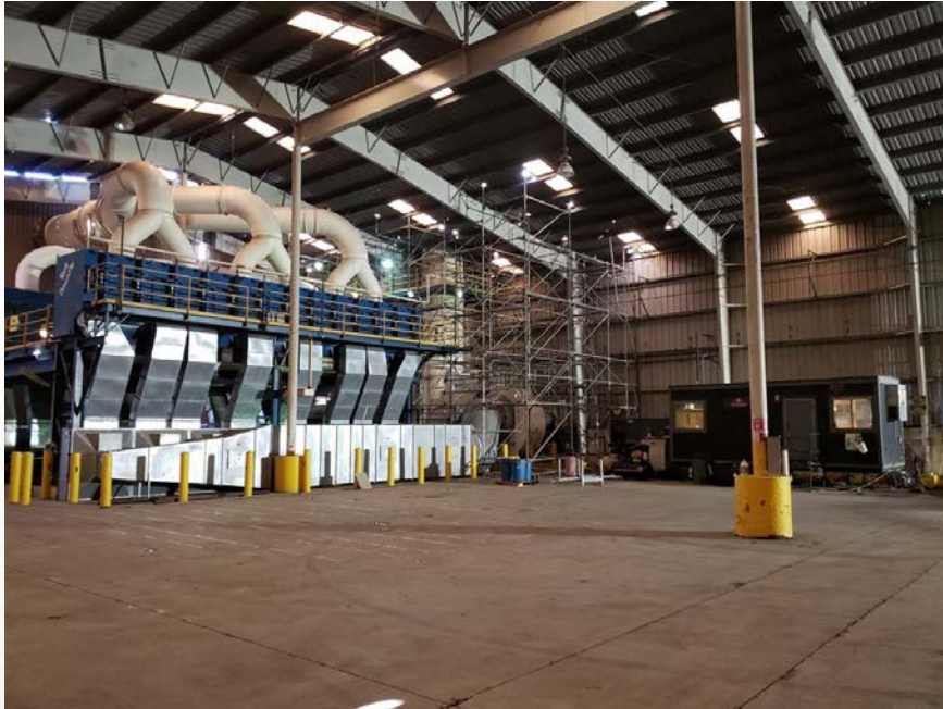
Torit Baghouse Units Decontamination and Deconstruction
