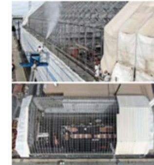
Smelter Building Segment 2 Full Enclosure Unit Takedown
