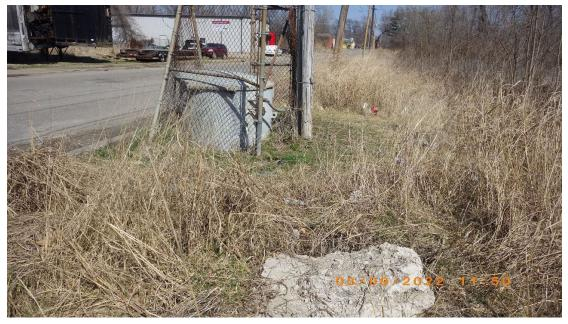
8: RIMG0048 Description: Concrete block covering open manhole. Location: On North 73<sup>rd</sup> Street, just south of the intersection with State Street. Date/Time: March 9, 2022, 11:50AM
