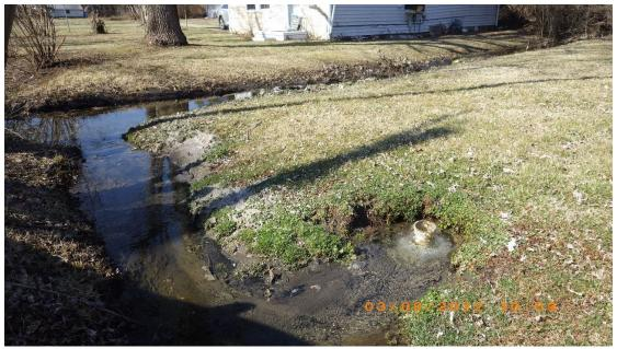
4: RIMG0044 Description: Active discharge of sanitary waste from cleanout. Location: North 82<sup>nd</sup> Street. Date/Time: March 9, 2022, 10:09AM
