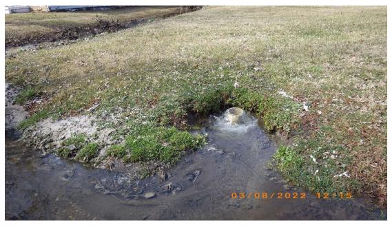
1: RIMG0041 Description: Active discharge of sanitary waste from cleanout. Location: North 82<sup>nd</sup> Street. Date/Time: March 8, 2022, 12:15PM
