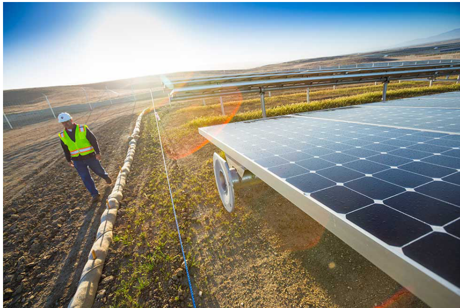
California Valley Solar Ranch in San Luis Obispo County. Photo credit: Bechtel .
