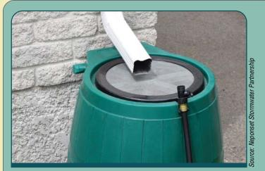
This residential rainbarrel incorporates a screen at the intake to keep out debris, mosquitoes and other creatures.
