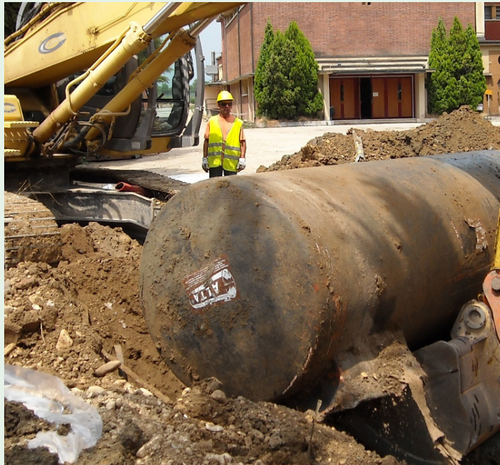
This abandoned gas station likely had or has five underground storage tanks, underground piping and five above ground vent pipes.
