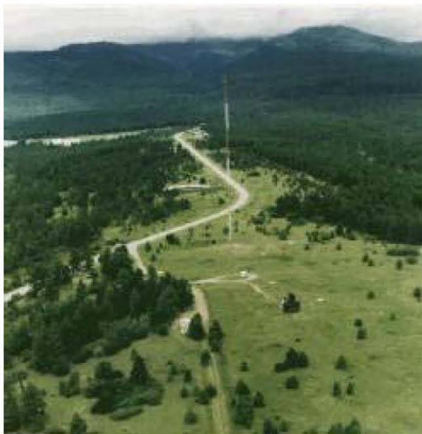
TA-06 Meteorological tower
