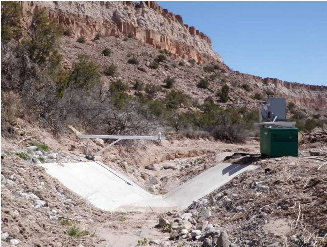
E060.1 Stream gage downstream view
