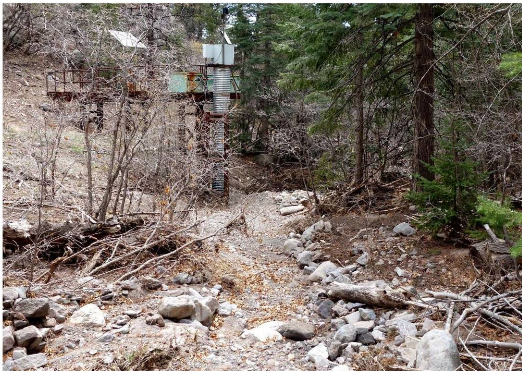
E240 Stream gage downstream view
