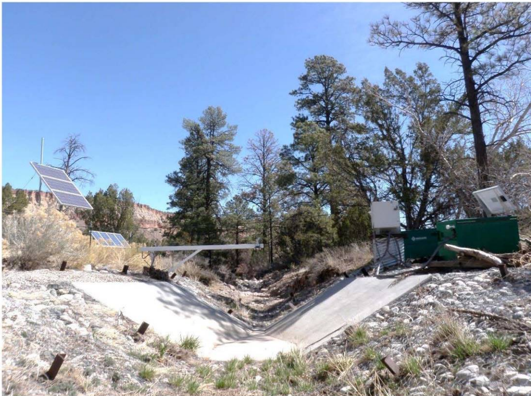
E050.1 Stream gage downstream view
