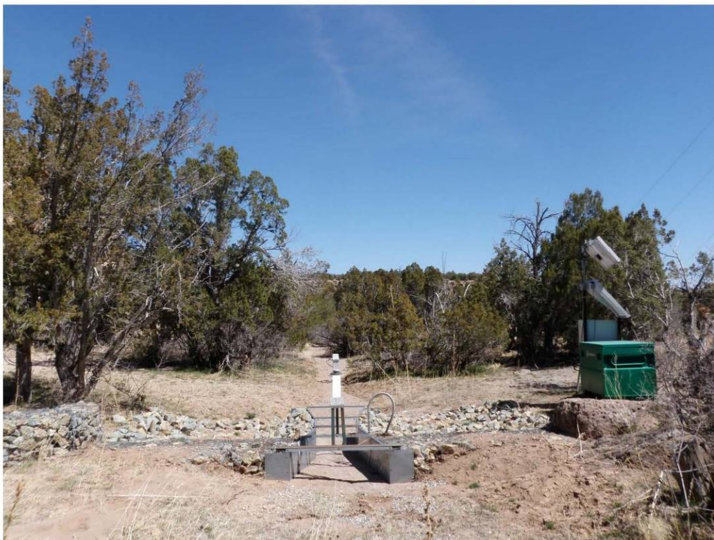
E229.3 Stream gage downstream view
