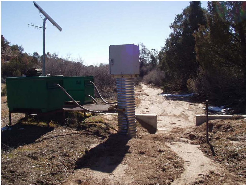
E267 Stream gage downstream view
