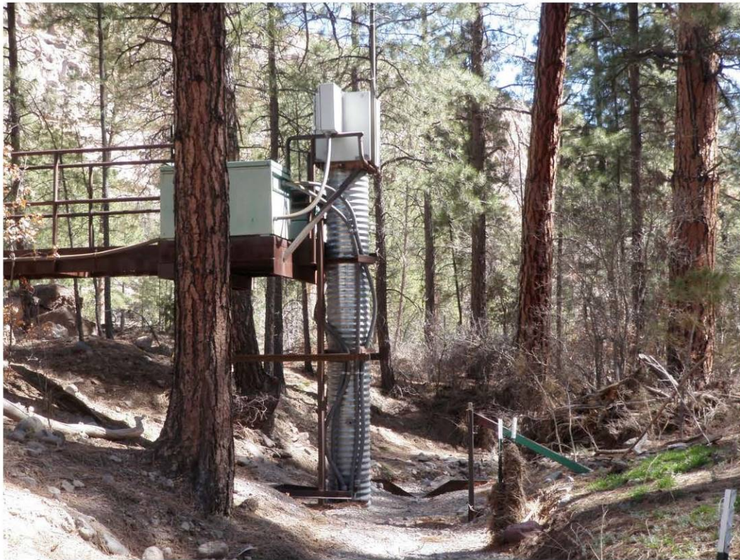
E030 Stream gage downstream view
