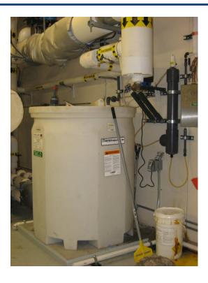
Photograph - NPDES-03A027-18-006 SCC Chiller Cooling Towers - Corrosion Inhibitor Feed Tank
