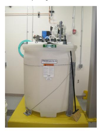
Photograph - NPDES-03A027-18-013 SCC Trinity Cooling Towers - pH Adjustment Chemical Feed Tank
