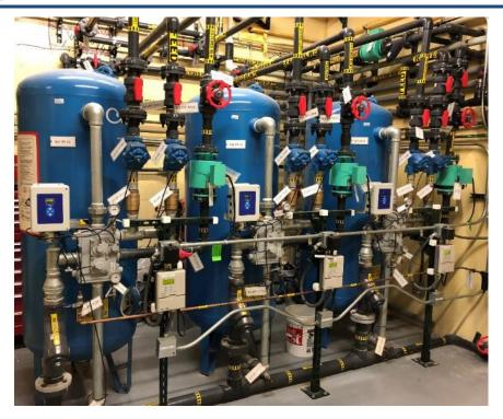
Photograph - NPDES-051-18-005 **Main LLW Treatment – Pressure Filters**
