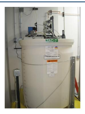
Photograph - NPDES-03A027-18-014 SCC Trinity Cooling Towers - Corrosion Inhibitor Feed Tank
