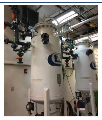
Photograph - NPDES-05A055-18-010 **HEWTF - Activated Carbon Filter Tanks**
