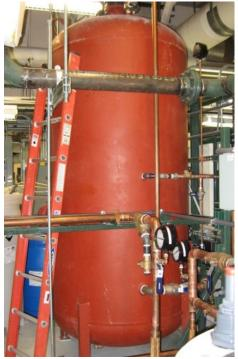
Photograph - NPDES-03A199-18-006 **LDCC Neutralization Tank**
