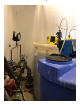
Photograph - NPDES-03A048-18-006 **TA-53-963 Cooling Towers Corrosion Inhibitor and De-Chlorination Feed Tanks**
