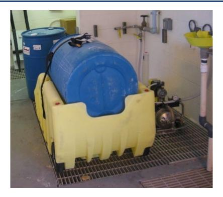
Photograph - NPDES-13S-18-016 SWWS Sludge Polymer Feed Tank
