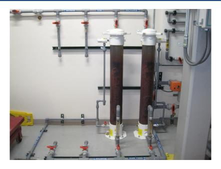
Photograph - NPDES-03A027-18-012 SCC Trinity Cooling Towers - Brominators
