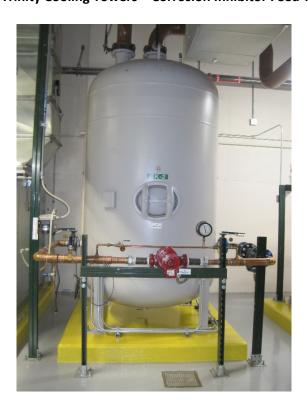
Photograph - NPDES-03A027-18-015 SCC Trinity Cooling Towers — Neutralization Tank
