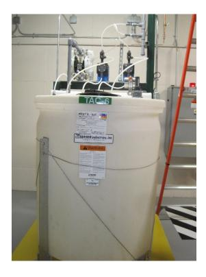
Photograph - NPDES-03A027-18-011 SCC Trinity Cooling Towers - Dechlorination Chemical Feed Tank
