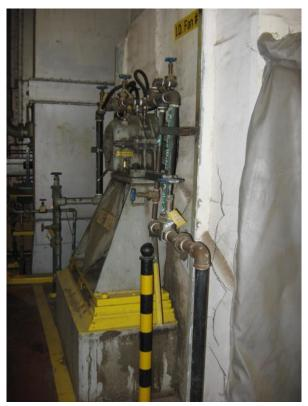
Photograph - NPDES-001-18-007 **Power Plant - Induced Draft Fan with Bearings Cooled by Cooling Tower Water**
