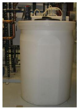
Photograph - NPDES-03A199-18-008 LDCC Dechlorination Chemical Feed Tank
