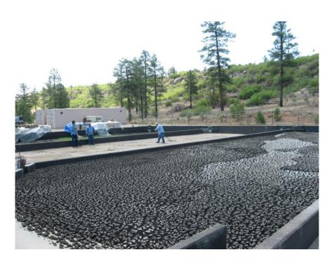
Photograph - NPDES-13S-18-020 SWWS Sludge Drying Beds
