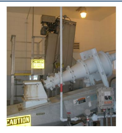
Photograph - NPDES-13S-18-007 SWWS Bar Screen at the Headworks
