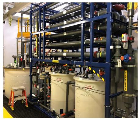
Photograph - NPDES-051-18-006 Main LLW Treatment - Microfilter
