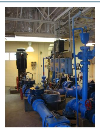
Photograph - NPDES-13S-18-018 SWWS Reuse Pumps and Chlorine Analyzer
