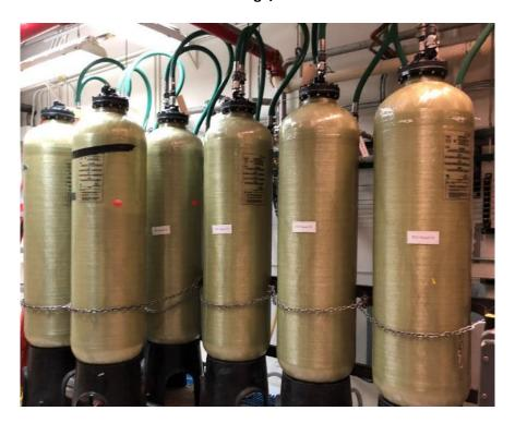
Photograph - NPDES-051-18-008 Main LLW Treatment – Ion Exchange Tanks
