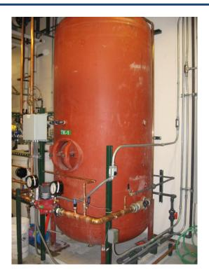
Photograph - NPDES-03A027-18-008 SCC Chiller Cooling Towers - Neutralization Tank
