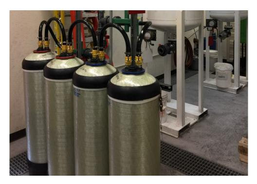
Photograph - NPDES-05A055-18-011 **HEWTF - Ion Exchange Tanks**
