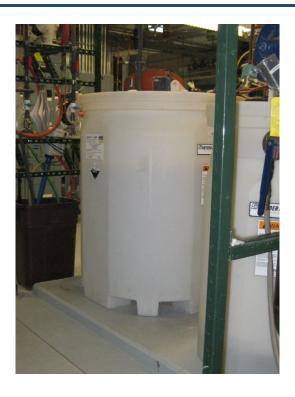
Photograph - NPDES-03A199-18-005 LDCC Corrosion Inhibitor and pH Adjustment Chemical Feed Tanks
