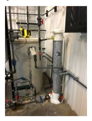
Photograph - NPDES-03A048-18-010 TA-53-978 Cooling Towers Brominator
