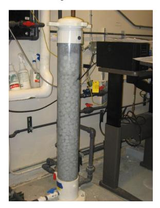
Photograph - NPDES-03A027-18-009 SCC Chiller Cooling Towers - Brominator
