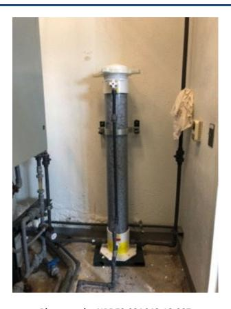
Photograph - NPDES-03A048-18-007 TA-53-963 Cooling Towers Brominator
