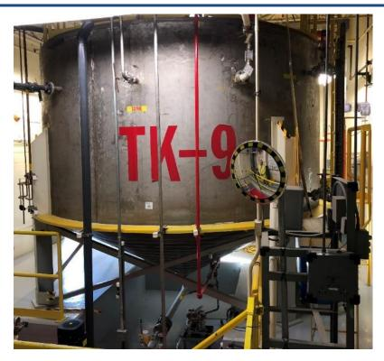
Photograph - NPDES-051-18-007 Main LLW Treatment – Ion Exchange/Reverse Osmosis Feed Tank TK9
