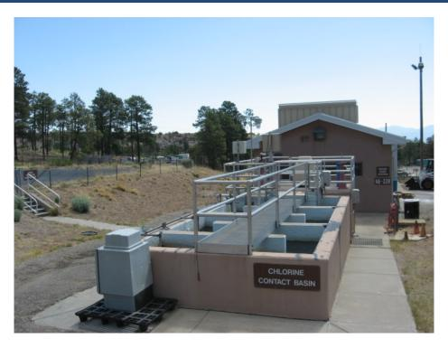
Photograph - NPDES-13S-18-014 SWWS Chlorine Contact Chamber
