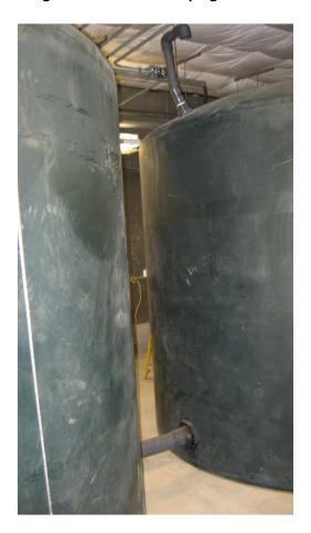
Photograph - NPDES-03A160-18-006 NHMFL Cooling Tower Blow Down Storage Tanks Prior to Discharge to Outfall 03A60 (inactive)
