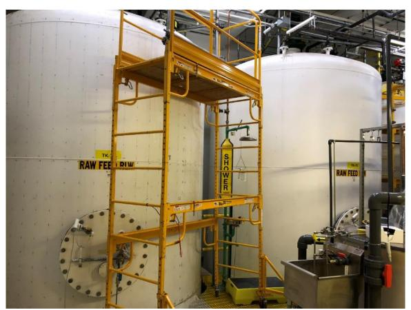
Photograph - NPDES-051-18-004 **Main LLW Treatment – Reaction Tanks**
