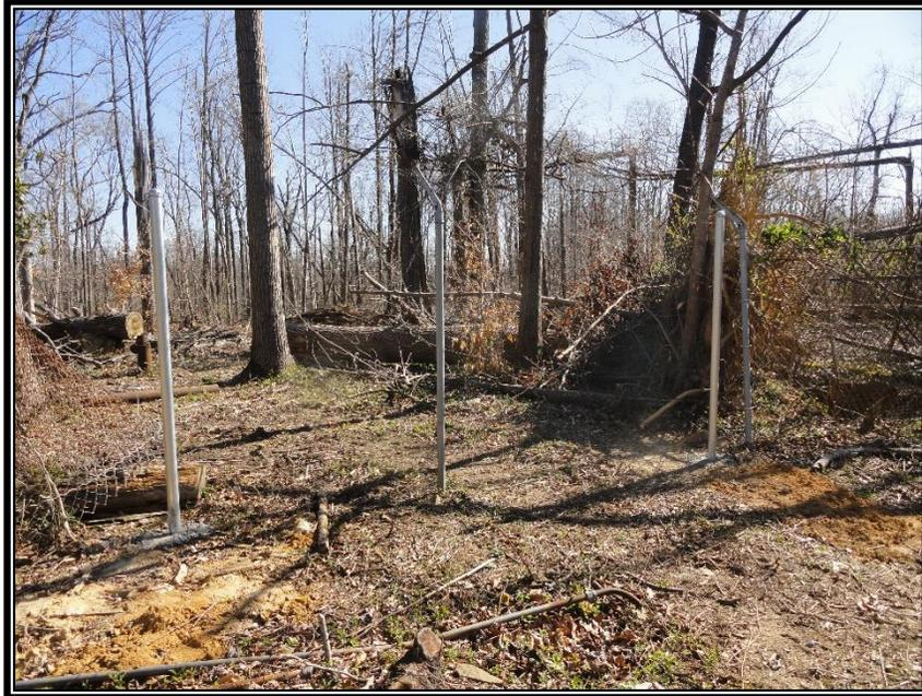
**Photograph No. 3:** Northeasterly view of the 12- to 16-foot gap in the Facility Security fence on March 29, 2022.
