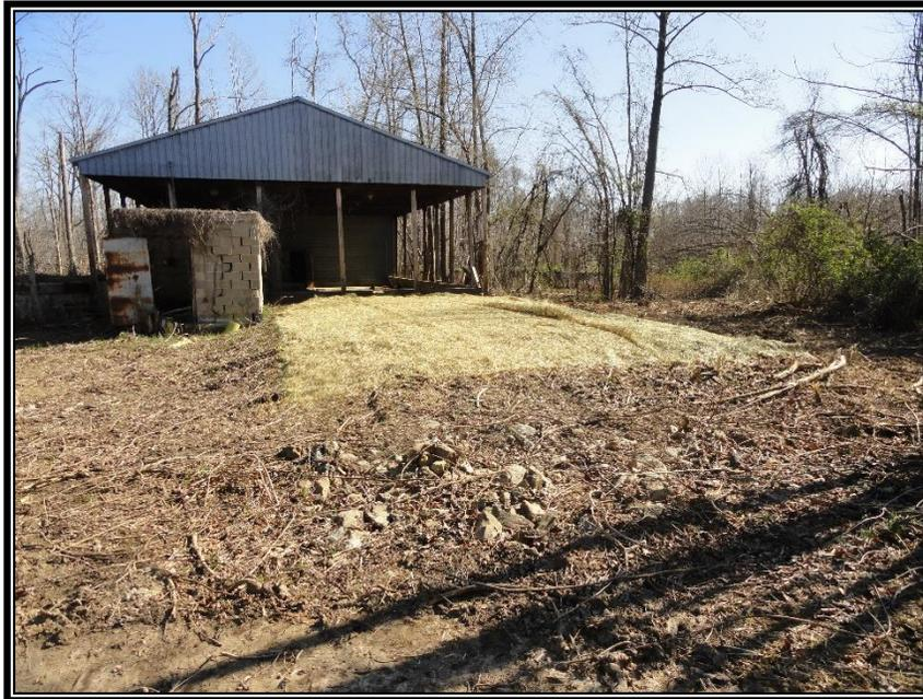
**Photograph No. 7:** Northeasterly view of the hazardous waste landfill cap on March 29, 2022, with erosion control blankets applied.
