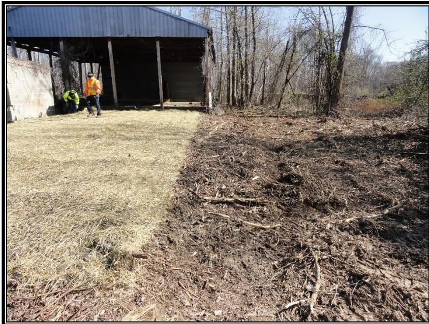
**Photograph No. 8:** Northern view of the hazardous waste landfill cap on March 29, 2022, with erosion control blankets applied.
