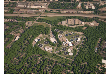
Nelson Wastewater Treatment Plant, Johnson County, Kansas
