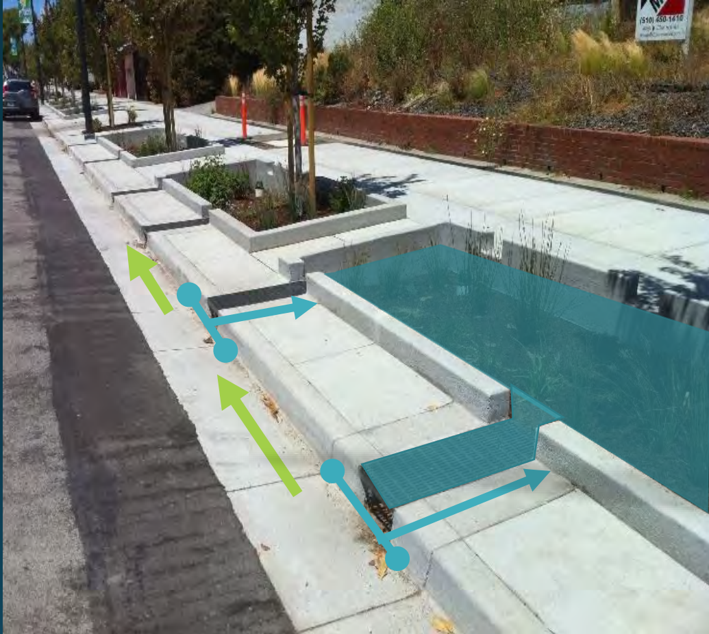
Off-line design with trench drains & wood mulch
