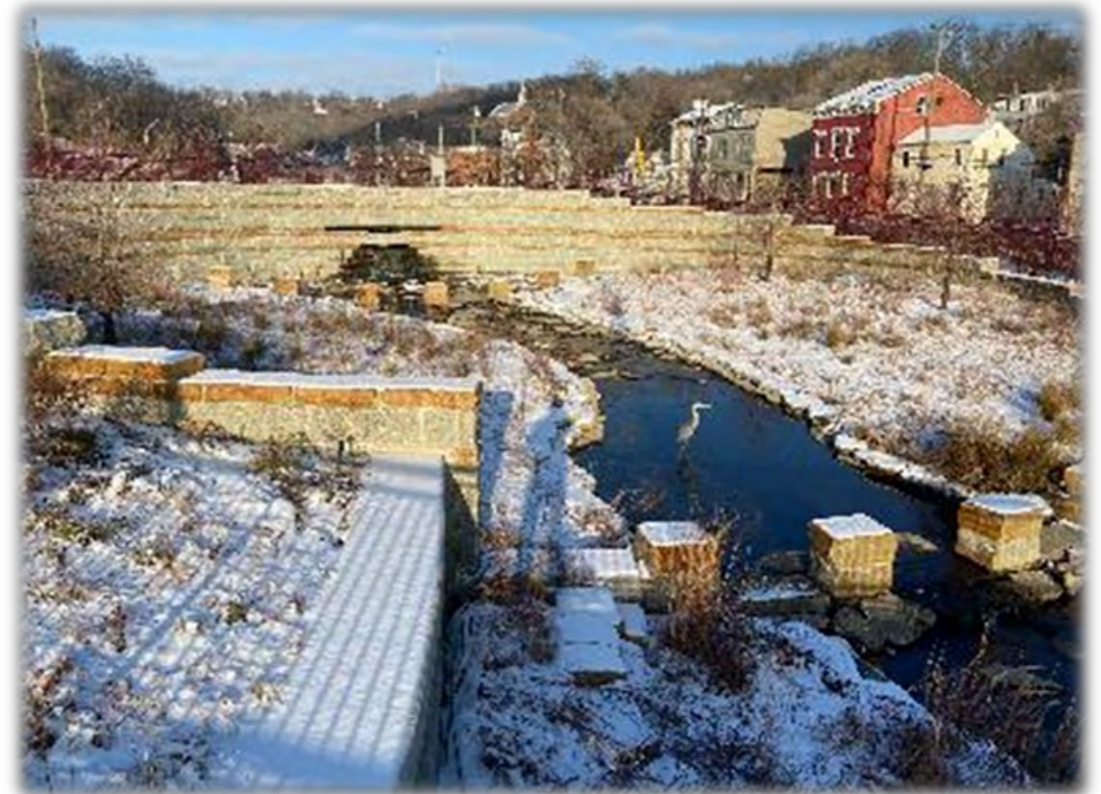
Lick Run Greenway Headwaters
