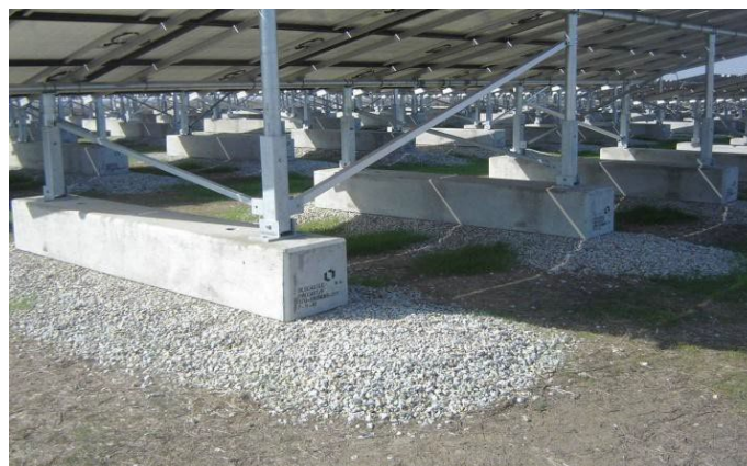
Figure 5-2: Precast ballast foundation for fixed tilt PV on a landfill.
