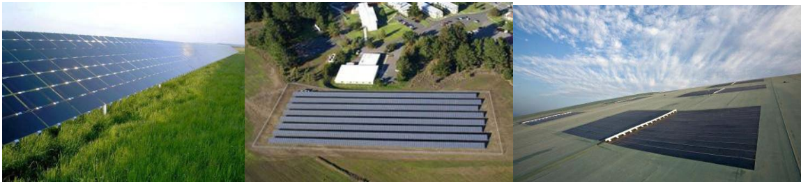
Figure 3-4: Thin-film solar modules installed on (i) solar energy cover and (ii/iii) fixed tilt mounting systems
