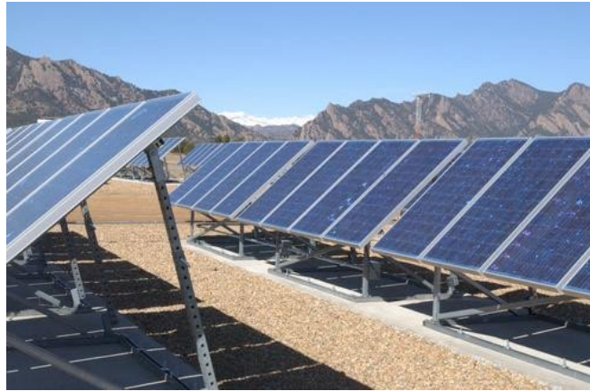
Figure 5-3: Slab foundation for PV system at Boulder, Colorado.
