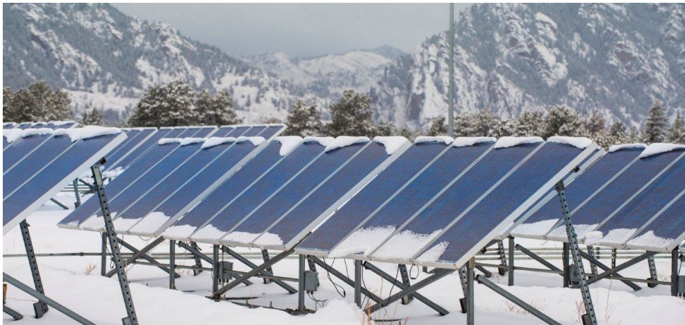
Figure 5-6: Snow loading on solar panels.
