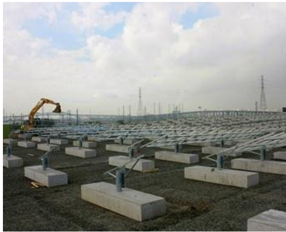
Figure 5-1: Ballasted anchoring system at Landfill 1A project at New Jersey Meadowlands.
