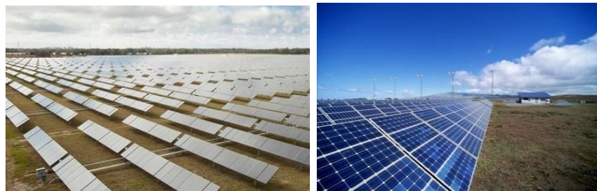
Figure 3-3: Mono- and multi-crystalline solar modules
