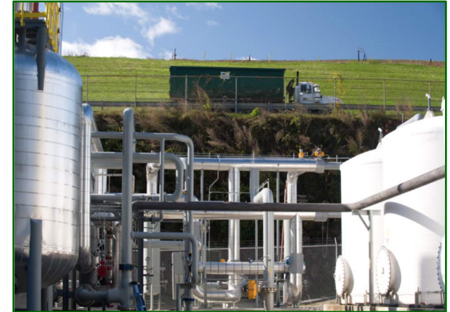
RNG Pipeline Project Rochester, NH
