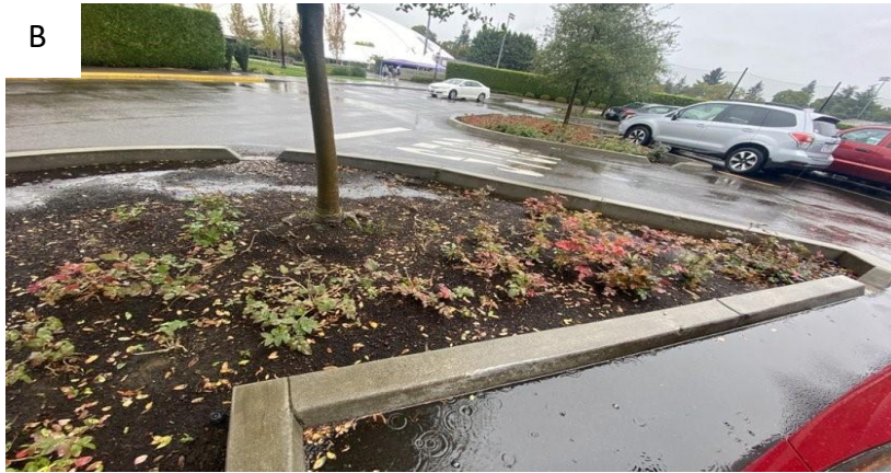
Figure 5. Current bioretention cell curb cutouts located in the Chiles parking lot create ponding and runoff; (A) Bio-cells short-circuiting; and (B) Stormwater runoff ponding outside of the bioretention cell.
