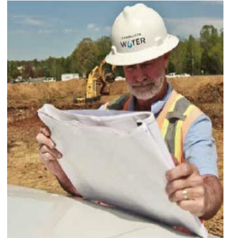
Reviewing engineering plans on site.
