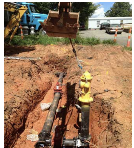
Installing new mains including a hydrant and valves.
