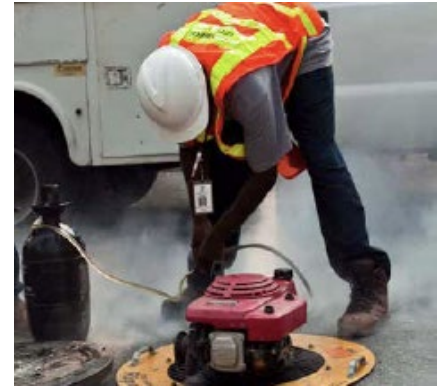
Worker performing maintenance on a sewer.
