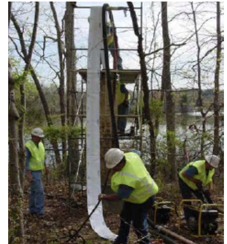
Workers prepare for pipe lining.
