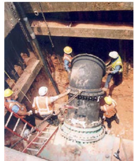
Installing a large diameter pipe fitting.
