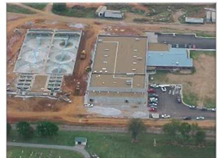
Treatment plant in Guthrie, KY that sells water to the LTRWC water systems.
