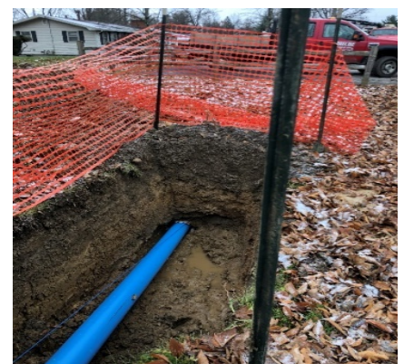
Tracing wiring surrounds the pit where the new pipe was laid.
