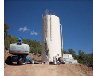
Figure 6. The new storage tank built to serve Ancones and El Llanito.
