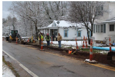
Figure 10. Installing water lines in the City of Sistersville. Source: https://www.tylerstarnews.com/news/local-news/2020/12/09/new-water-lines-being-installed-in-sistersville/
