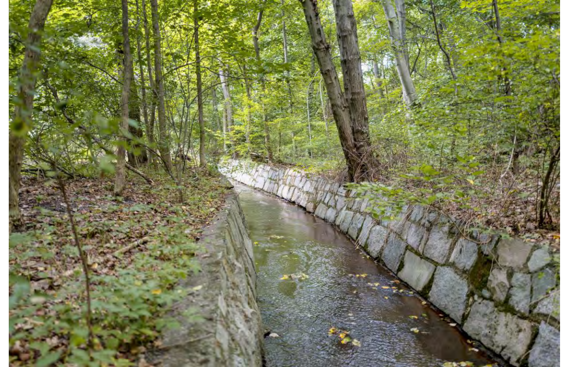
A portion of the Blackstone Canal – created from and near the River to transport goods through 49 locks
