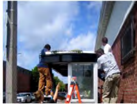
Green Roofs on Fairmount Line Bus Shelters
