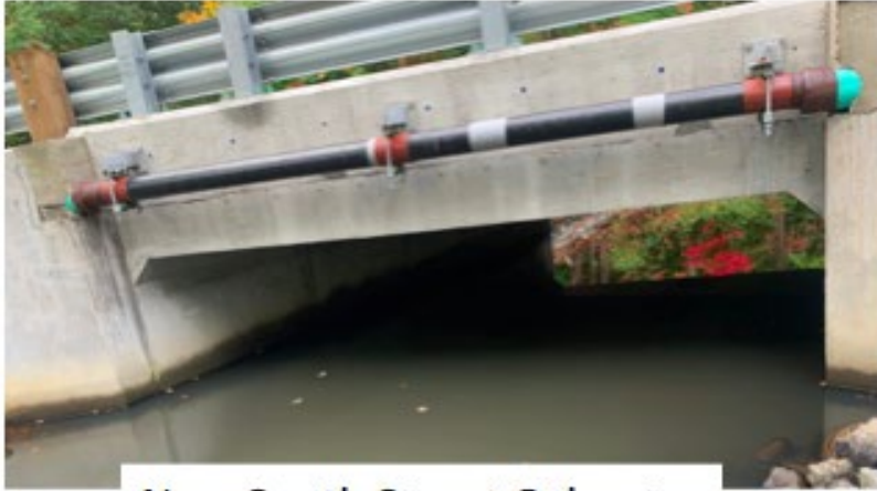
New South Street Culvert
