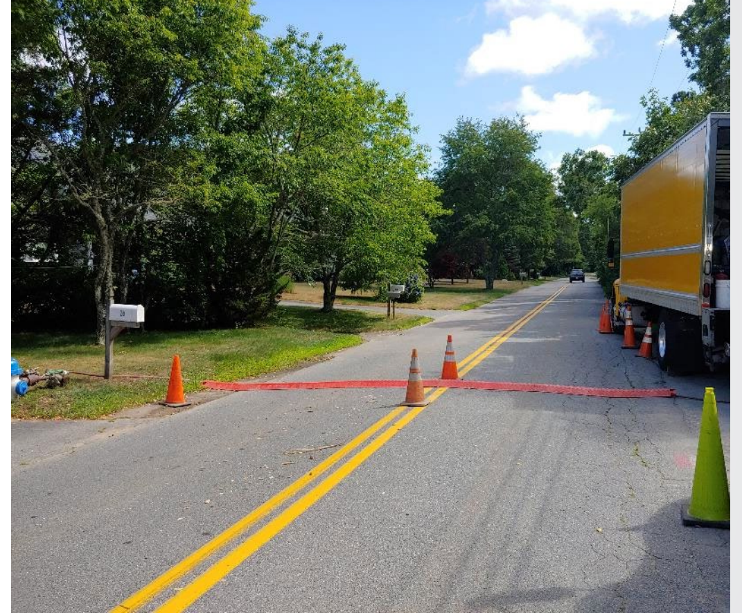
Water from hydrant with hose ramps to cross the road
