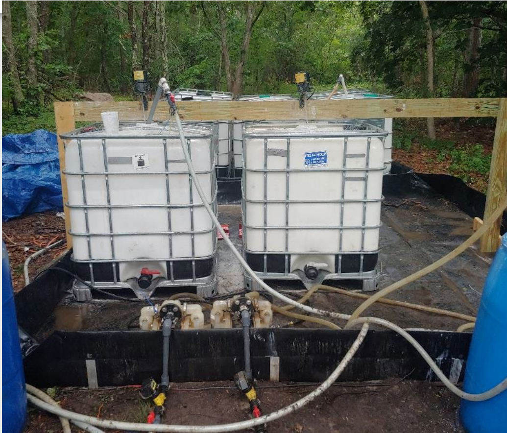
EVO Storage and Batching within secondary containment
