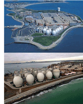
A view of Boston's Deer Island Wastewater Treatment Plant's redesigned facility
