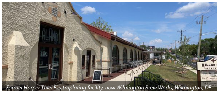
Former Harper Thiel Electroplating facility, now Wilmington Brew Works, Wilmington, DE
