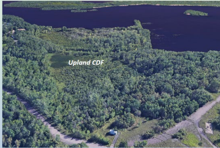
Before: Aerial view of Upland CDF area facing toward Spirit Lake pre-construction.
