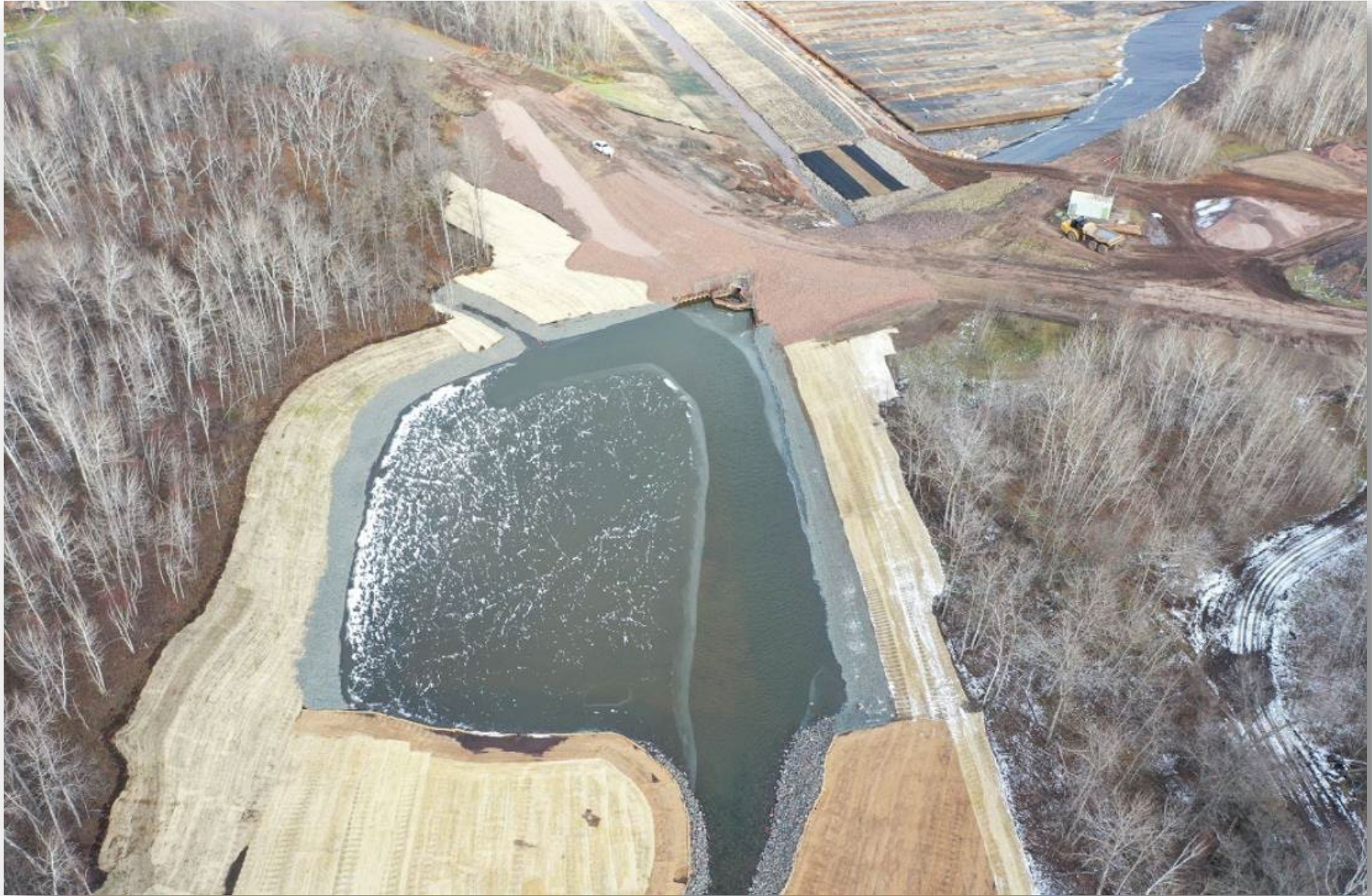
Weir Pond (Nov 2021)
