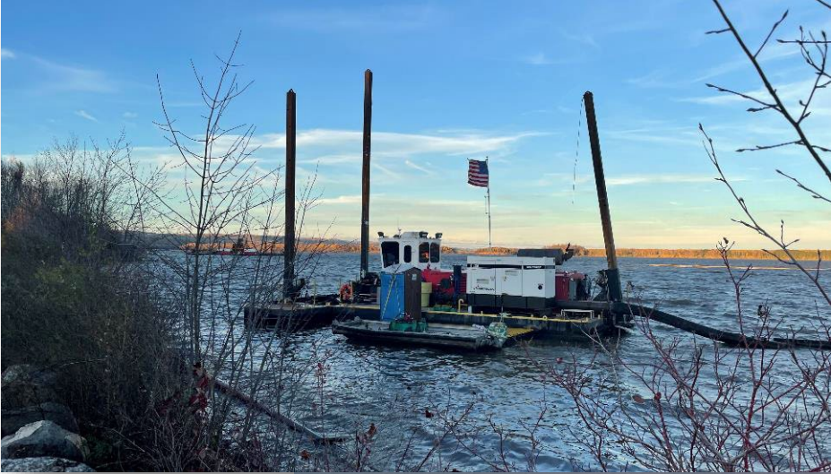
Hydraulic dredge sits on a barge in the Wire Mill Delta.
