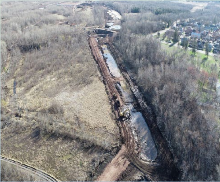
Before: Photograph of Upland CDF facing toward Spirit Lake in early construction stages.
