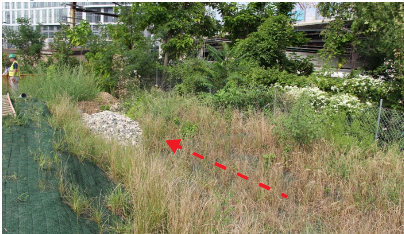
Figure 15-8. View of the area draining to the check dam.
