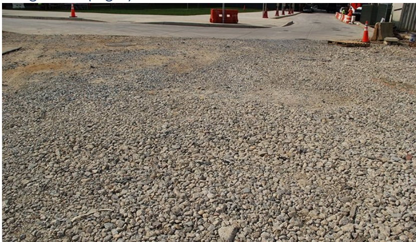
Figure 10-4. View of stone aggregate on the stabilized construction entrance.
