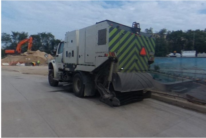
Figure 8-4. Street sweeper on Main Street, near the construction entrance.
