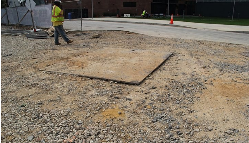
Figure 10-3. Metal plate on the construction entrance that covers buried utilities.
