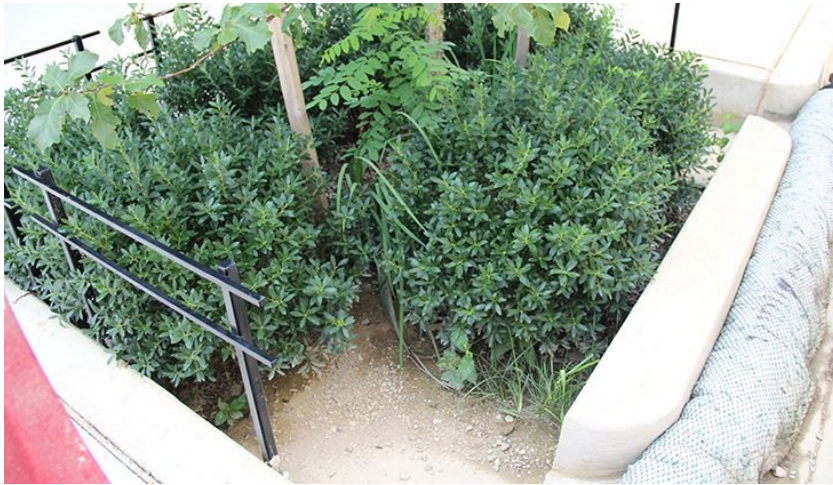
Figure 19-5. View of sediment accumulation in bioretention cell.
