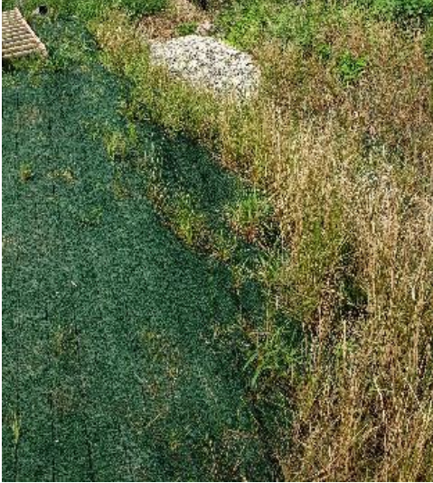
Figure 15-5. View of erosion control matting on the diversion berm.
