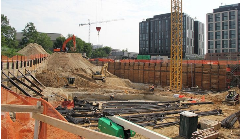
Figure 17-4. View of the active construction area.
