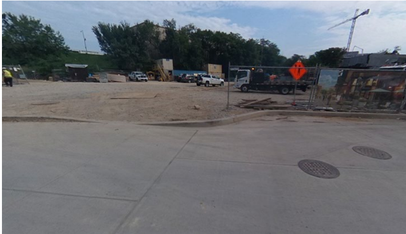
Figure 9-5. View of construction entrance on Main Street.
