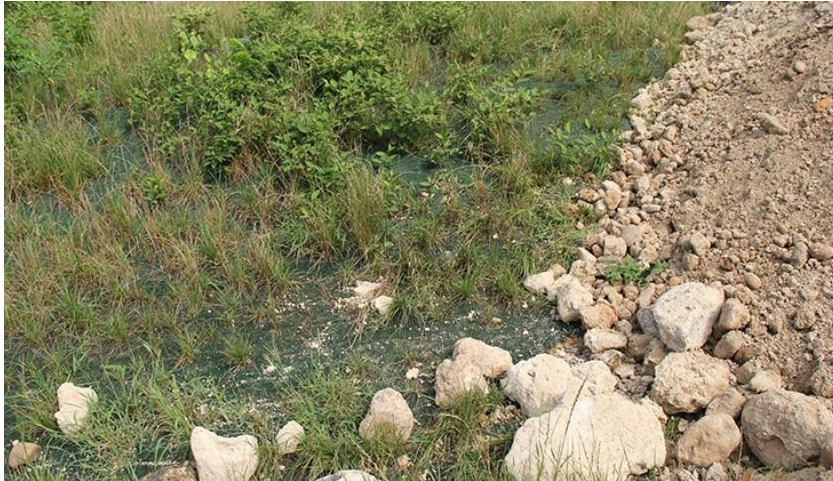
Figure 14-5. View of erosion control matting and vegetation on the slope adjacent to the soil stockpile.
