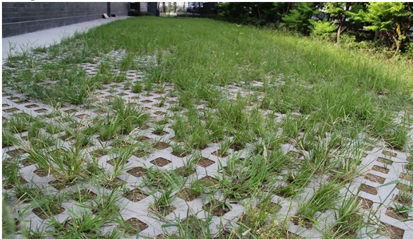
Figure 17-7. View of permeable pavers behind the parking garage.
