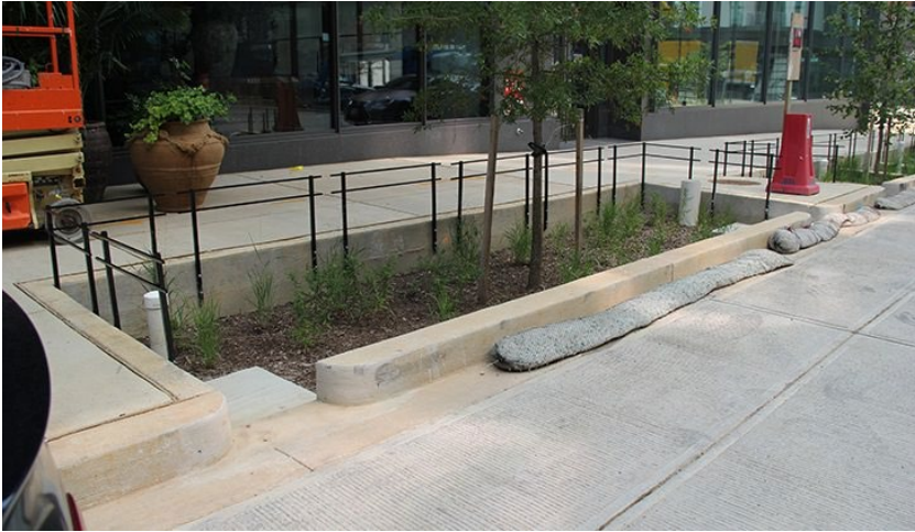
Figure 23-4. View of a third bioretention cell along First Street.
