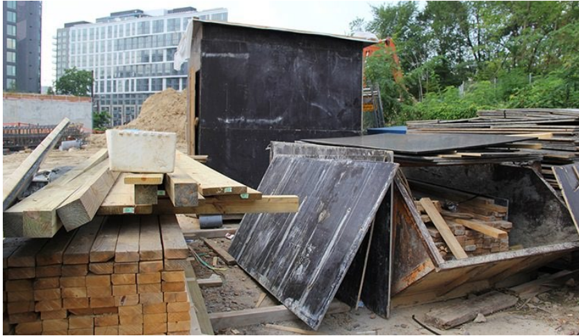
Figure 11-6. View of one side of the materials storage area.
