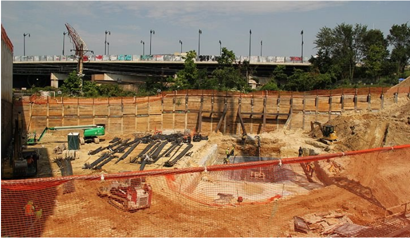
Figure 2-6. View the active construction area.
