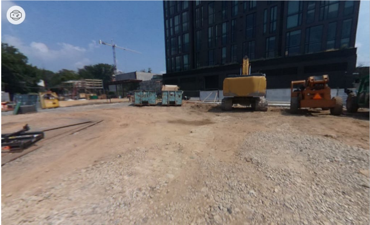
Figure 4-1. Starting view for Site 1, Area 21.
