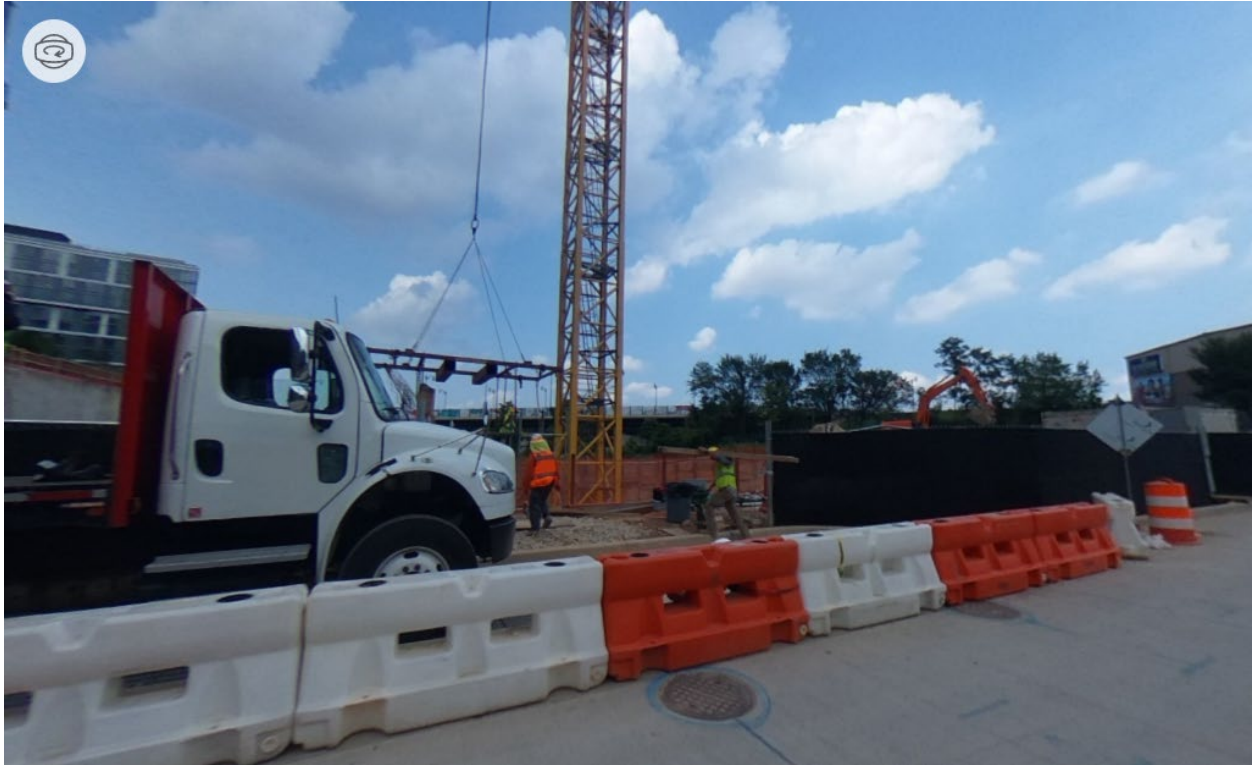
Figure 2-1. Starting view for Site 1, Area 19.
