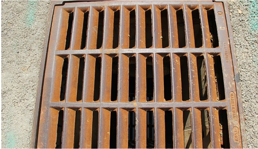
Figure 16-5. Close-up view of storm drain on Second Street.
