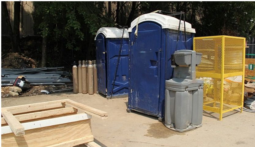
Figure 11-4. Portable toilets in the materials storage area.
