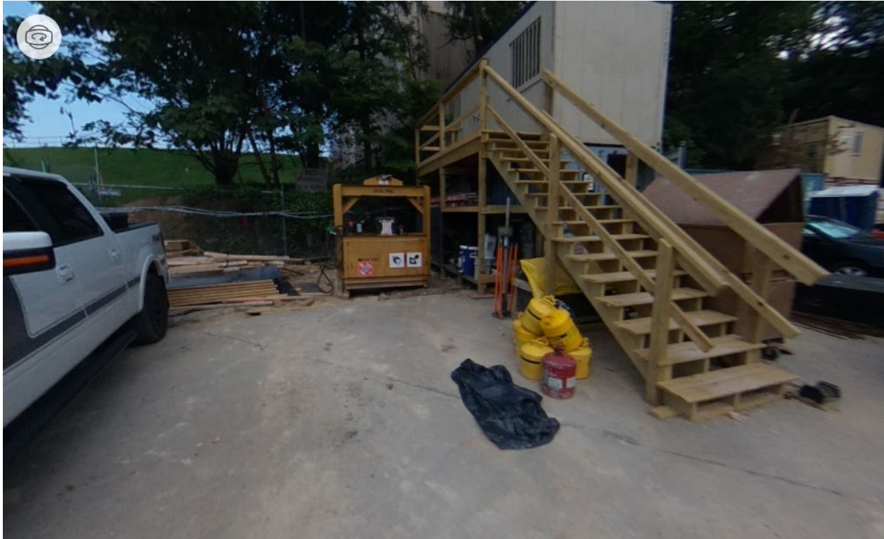
Figure 6-1. Starting view for Site 1, Area 23.
