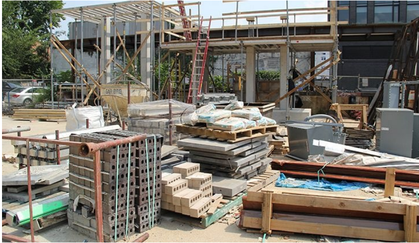
Figure 11-5. View of various construction materials stacked in the materials storage area.
