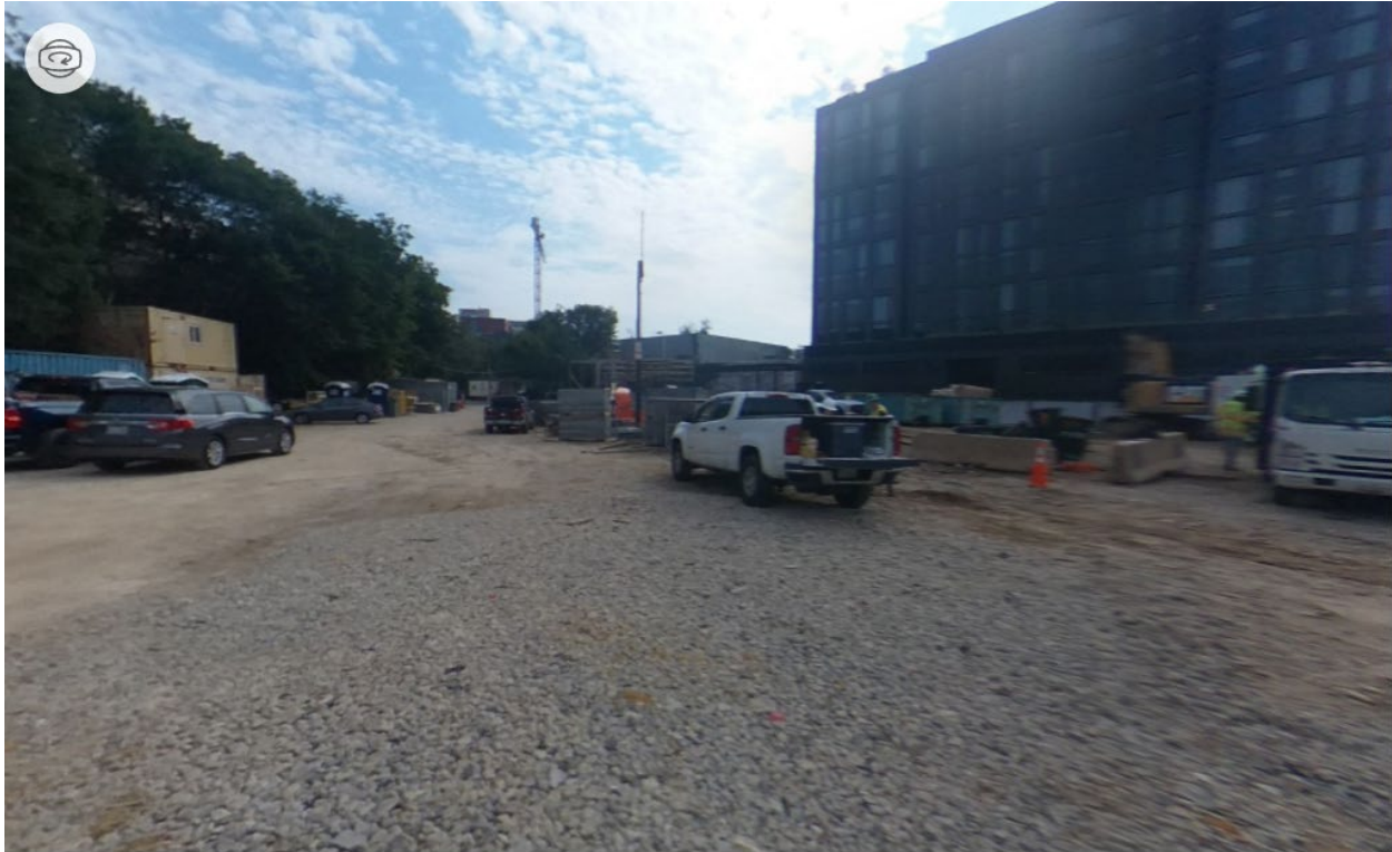
Figure 3-1. Starting view for Site 1, Area 20.
