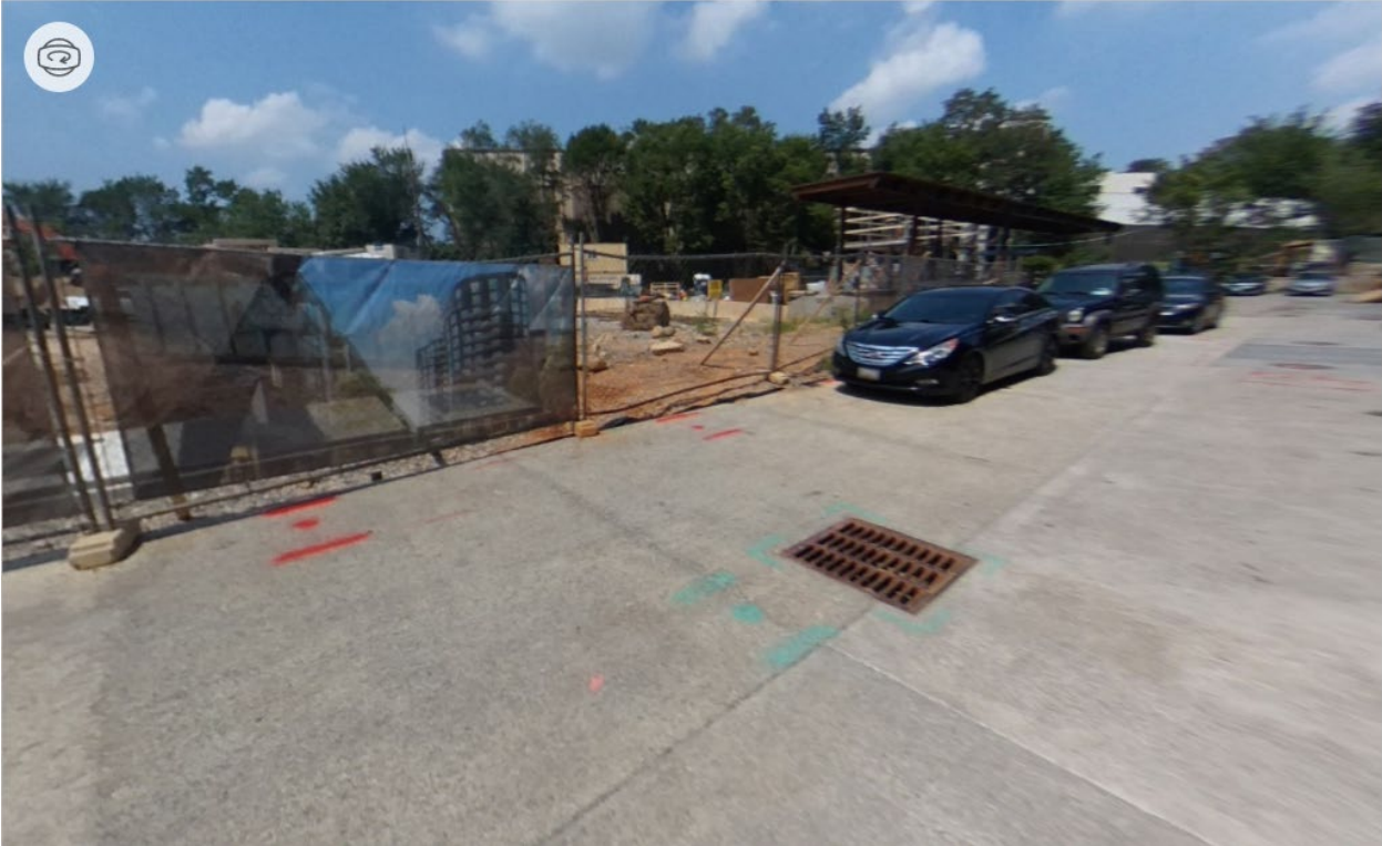
Figure 16-1. Starting view for Site 1, Area 33.
