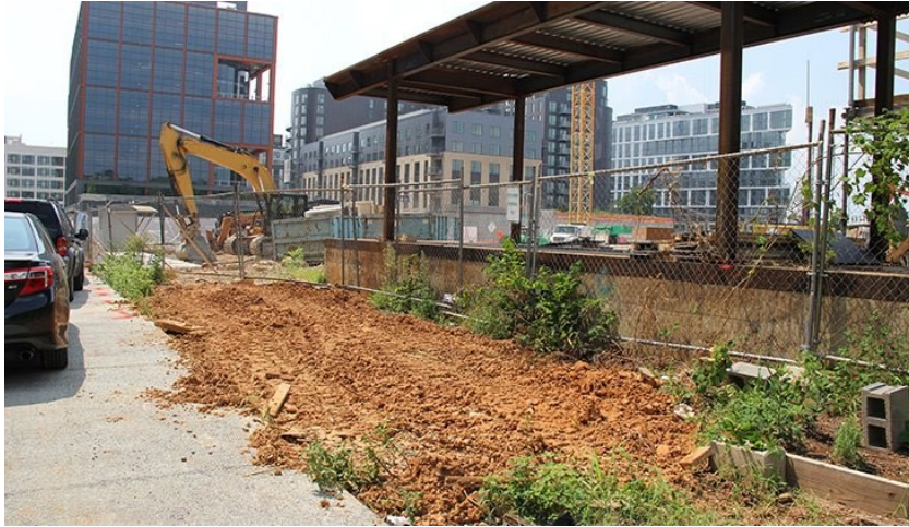
Figure 15-4. View of freshly disturbed area along Second Street.
