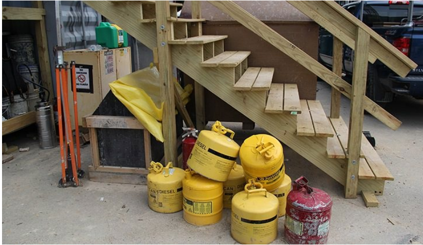
Figure 7-6. Pile of fuel containers near subcontractor's trailer.
