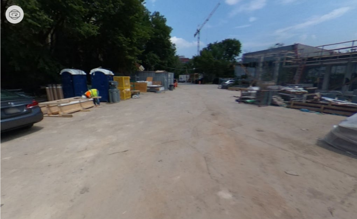
Figure 11-1. Starting view for Site 1, Area 28.
