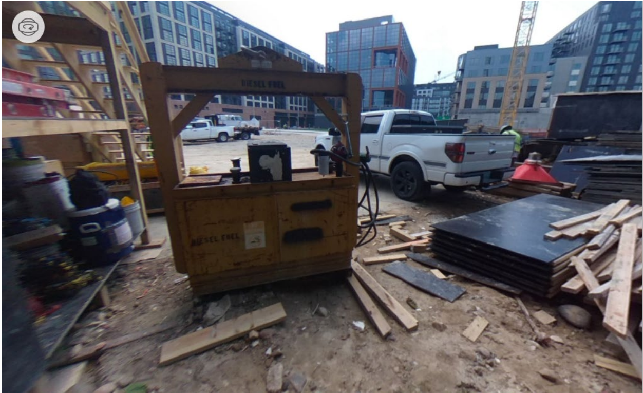
Figure 8-1. Starting view for Site 1, Area 25.
