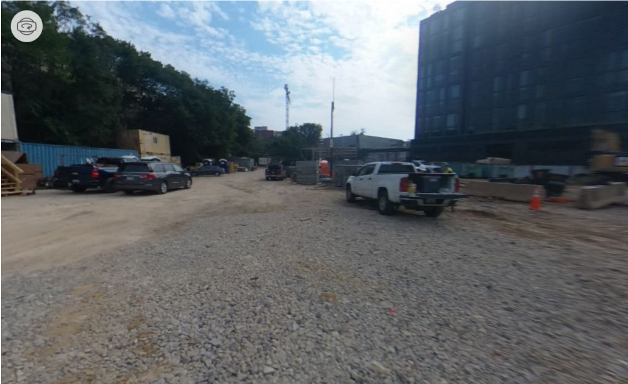
Figure 5-1. Starting view for Site 1, Area 22.
