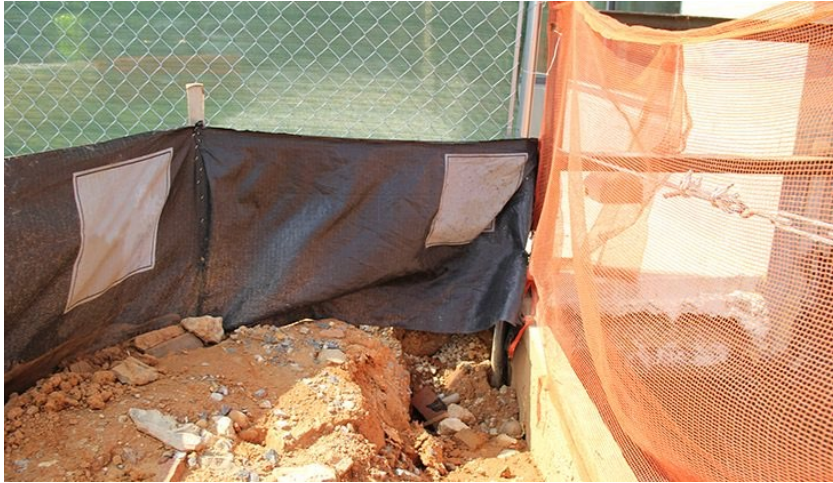
Figure 2-4. View of the silt fence in the area behind the truck.
