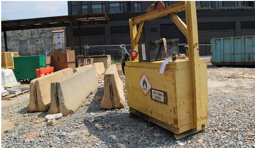
Figure 4-5. View of the back of the fuel tank.
