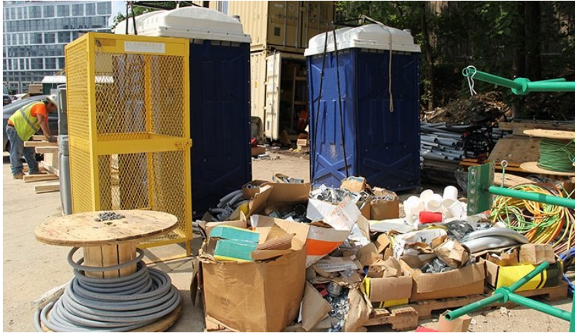
Figure 12-3. Pallet of construction materials behind the portable toilets.
