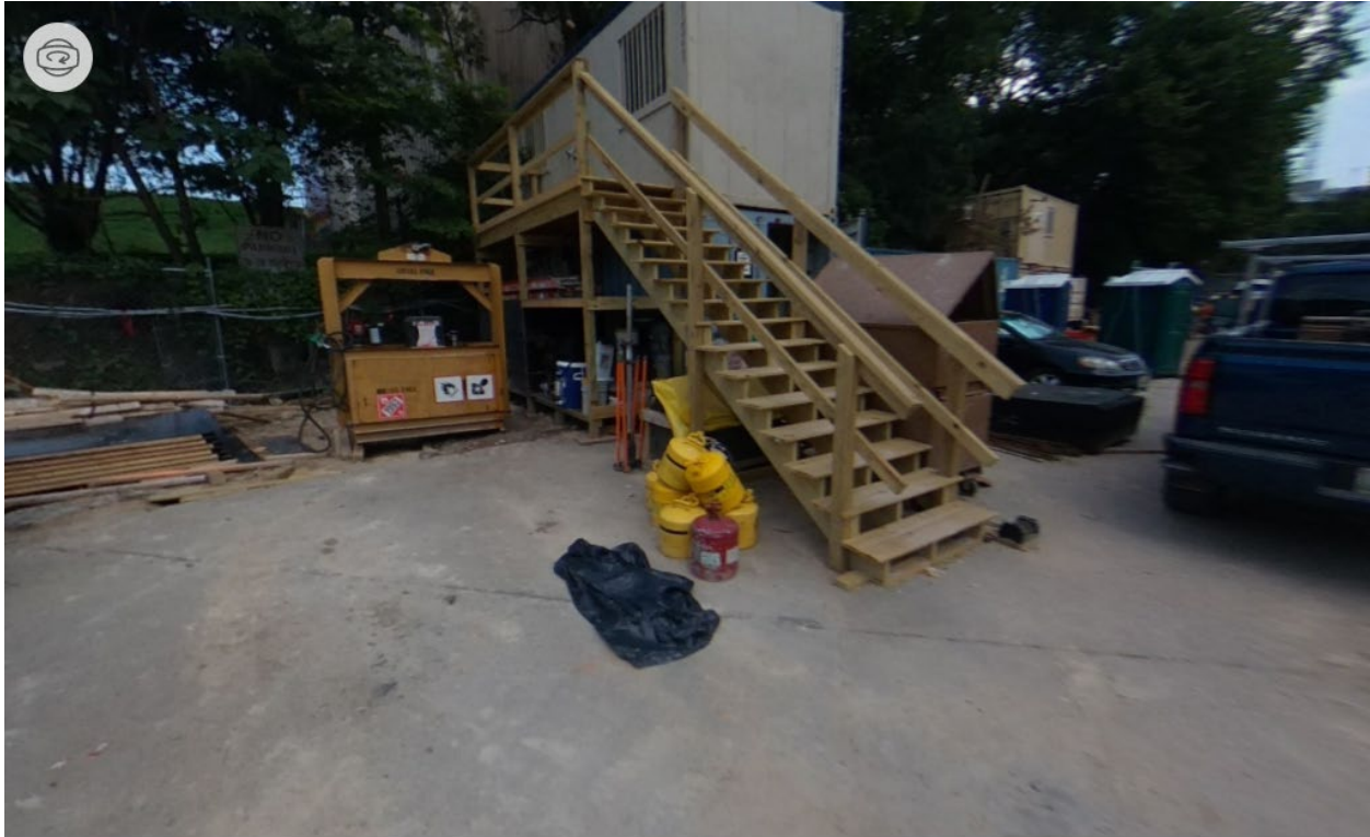
Figure 9-1. Starting view for Site 1, Area 26.
