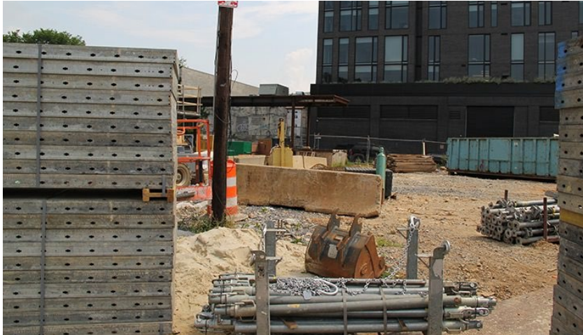
Figure 10-3. View of various building materials in the materials storage area.
