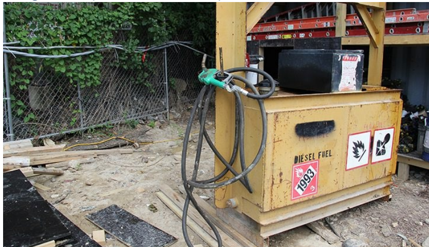
Figure 7-3. Fuel tank near subcontractor's trailer.
