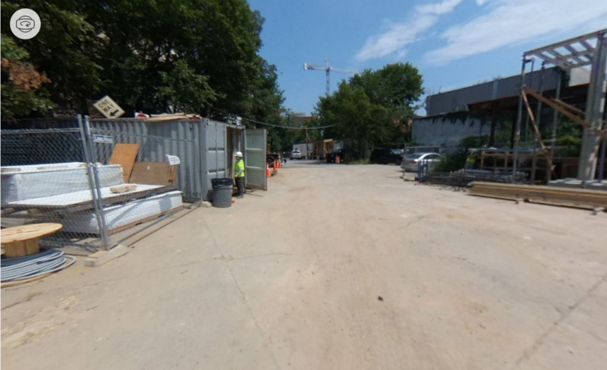
Figure 12-1. Starting view for Site 1, Area 29.
