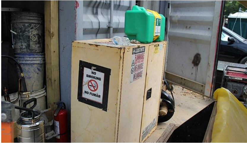
Figure 7-4. Flammables cabinet near subcontractor's trailer.
