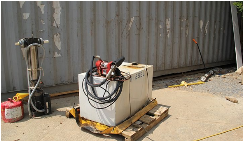
Figure 13-4. Fuel tanks by a trailer near the end of the materials storage area.
