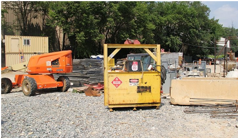
Figure 4-4. Fuel tank in the materials storage area.
