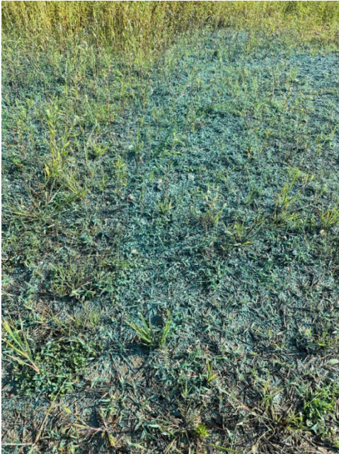
Figure 10-5. Close-up view of hydroseeding on the large stockpile.
