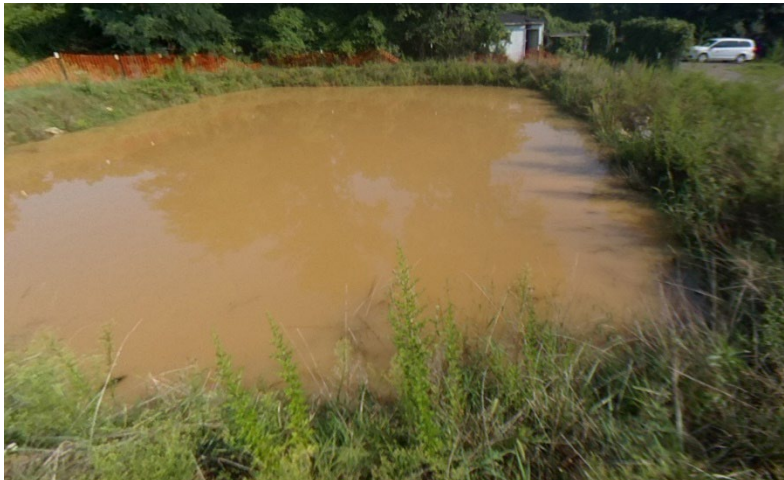
Figure 5-4. View of sediment trap full of turbid water.
