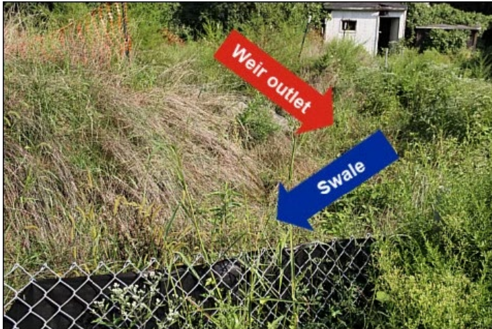
Figure 7-4. View of the sediment trap's outlet and downstream swale.
