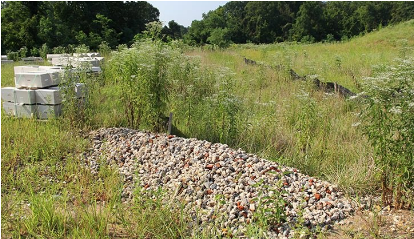
Figure 12-4. Check dam at the upgradient end of the grass swale.
