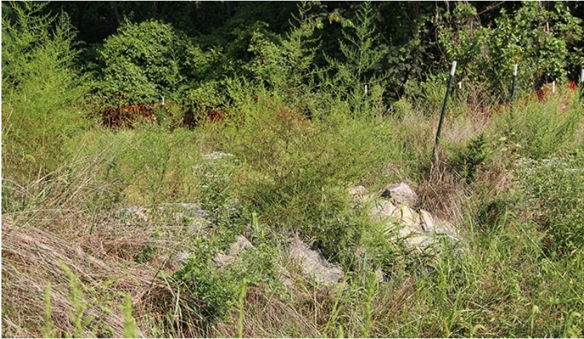
Figure 5-5. View of stone outlet on southern embankment of sediment trap.
