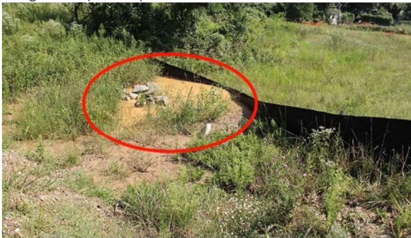
Figure 9-5. View of water ponded against the silt fence at the base of the large stockpile.
