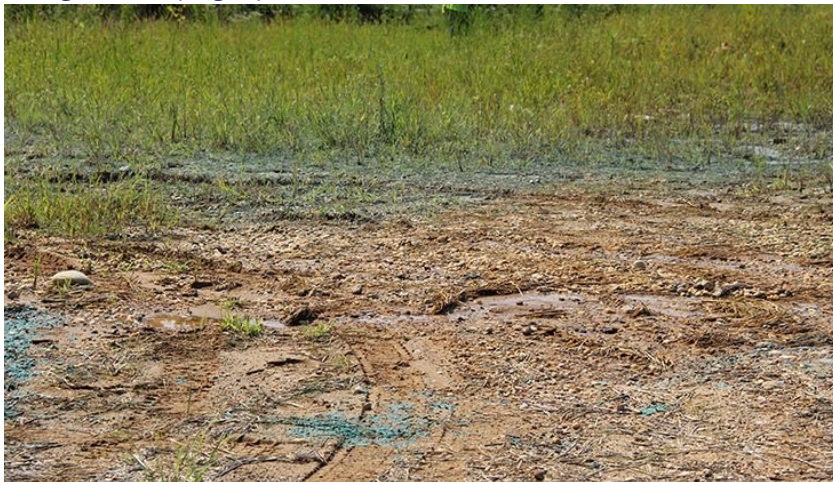
Figure 12-6. View of bare area adjacent to the construction entrance.
