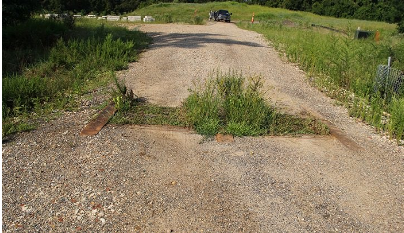
Figure 4-4. View of wash rack in the stabilized construction entrance.
