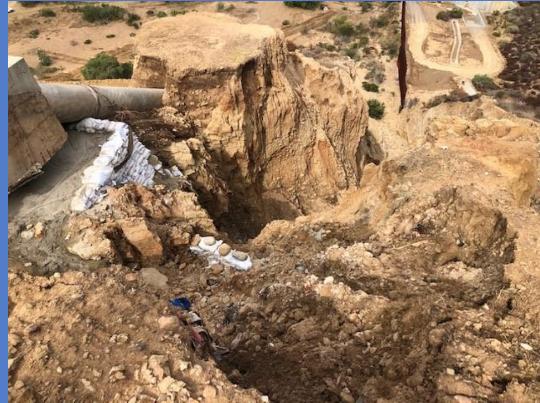
Ongoing Stabilization of PB-1A 8/3/2022
