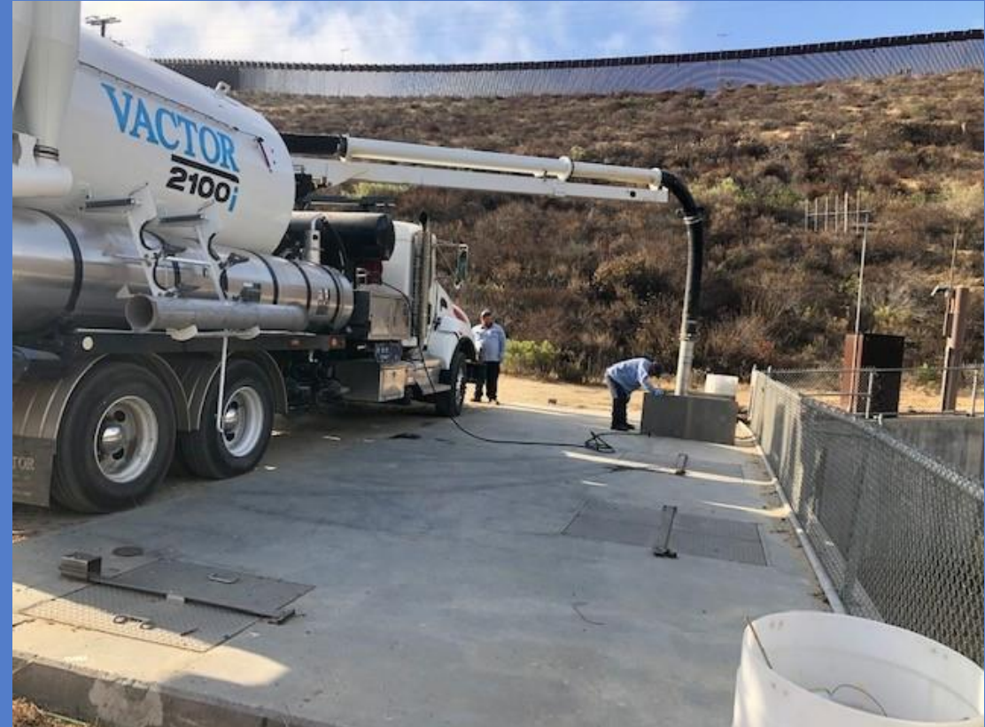
Sediment Removal at Smuggler's Gulch: 8/1/2022
