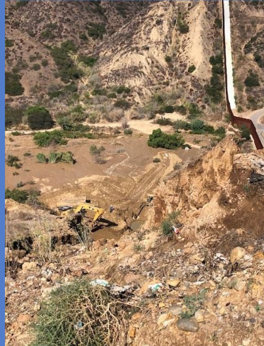
Slope Repair PB1B: 8/2/2022
