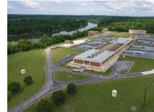
Photo credit: Metro Water Services
