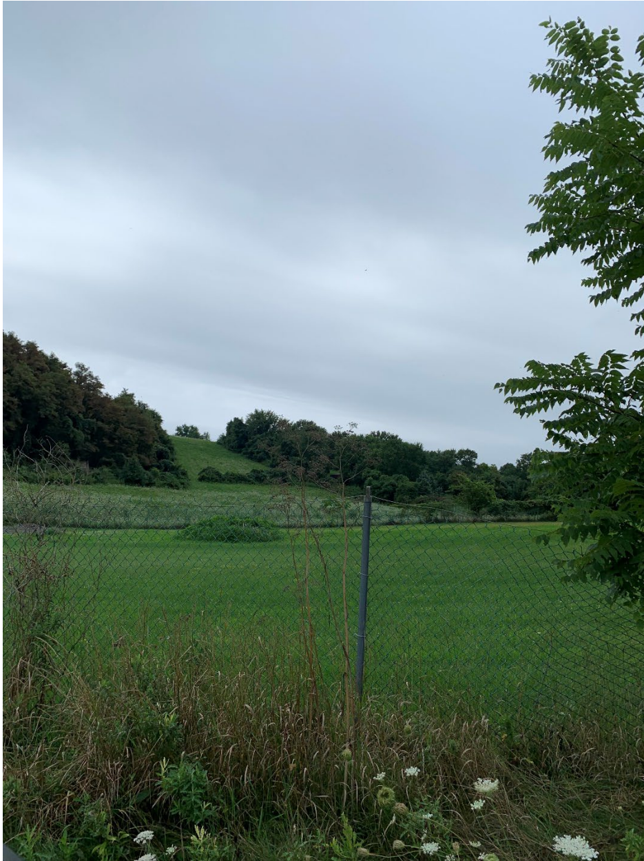
Picture 6: Facility Berm Facing Southwest
