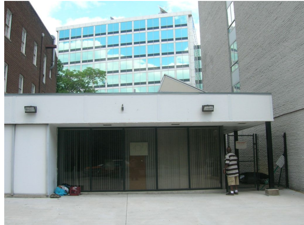
District's CAMP station
